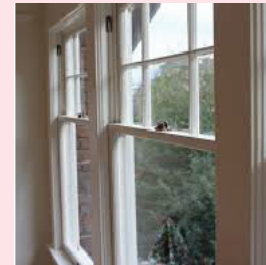
Paint on double-hung windows
