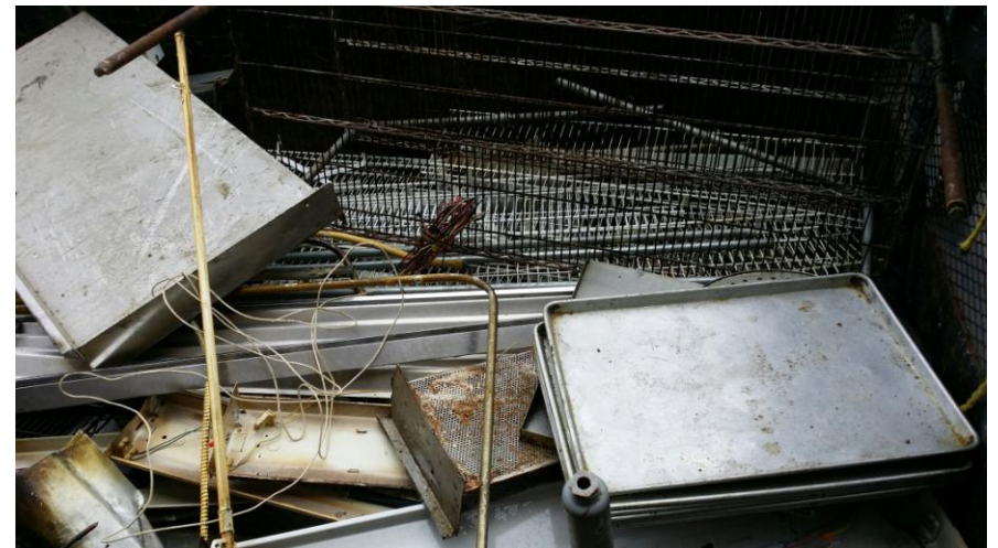
KITCHEN DEMO AND NEW PLACEMENT OF SINKS
