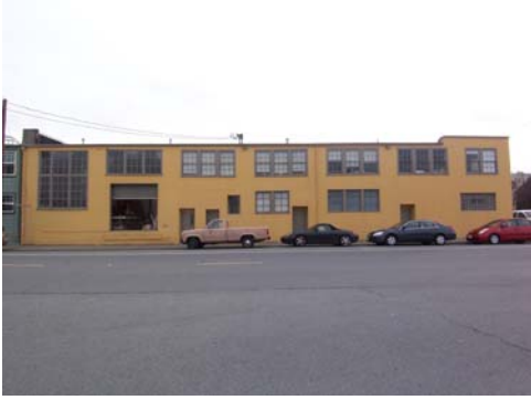
100_1950.JPG. 11/16/07, view to S
