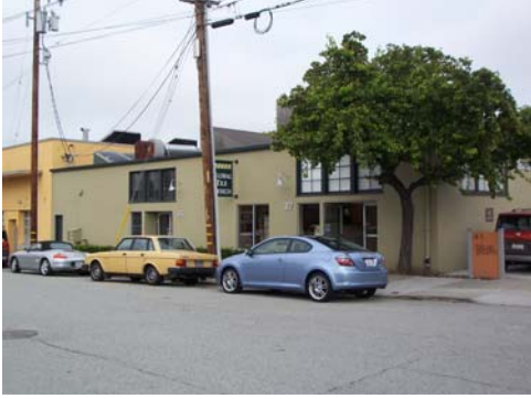
100_1955.JPG, 11/16/07, view to NE
