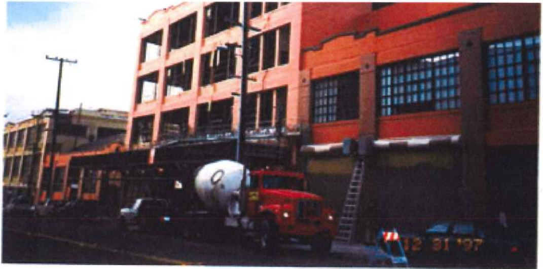
Below: BAVC's location at 2727 Mariposa St., undergoing renovations
