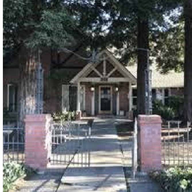
Progress Sonoma ADU 2007
