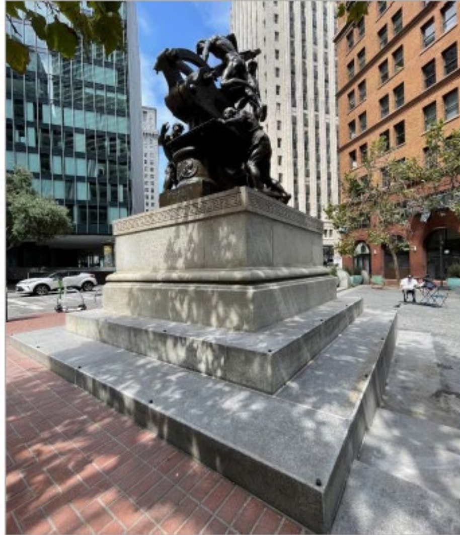
Image 56: Detail of areas the Mechanics monument after treatment.
