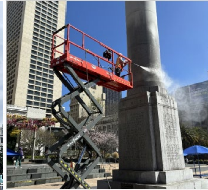
Image 3: Conservator rinsing the affected area with hot pressurized water from a scissor lift.
