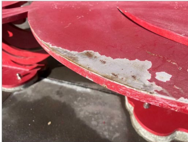
Image 3: Detail view of the red bench showing exposed primer, steel, and corrosion.
