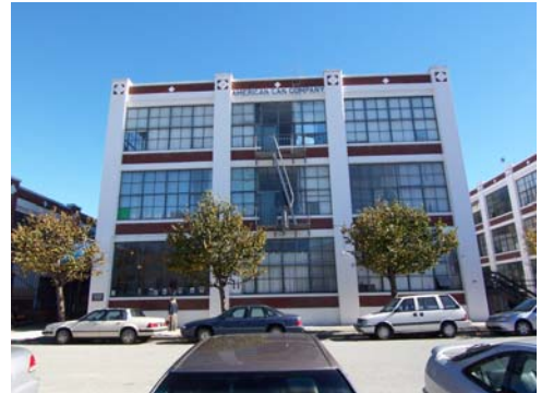
100_5726.JPG, 11/20/2007, view to E
