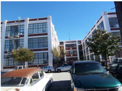
100_5727.JPG, 11/20/2007, view to E
