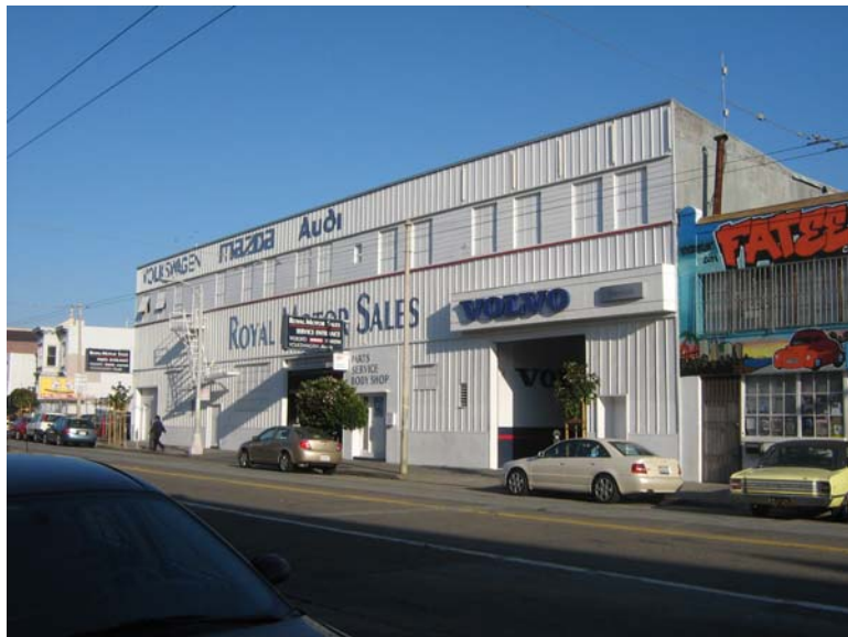
West façade of 1525 Howard Street (alternate address of 160 Kissling Street). Source: Page and Turnbull
