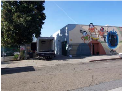
100_6479.JPG, 11/29/07, view to W, loading dock
