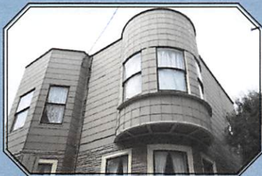
Before the Teevan Restoration
