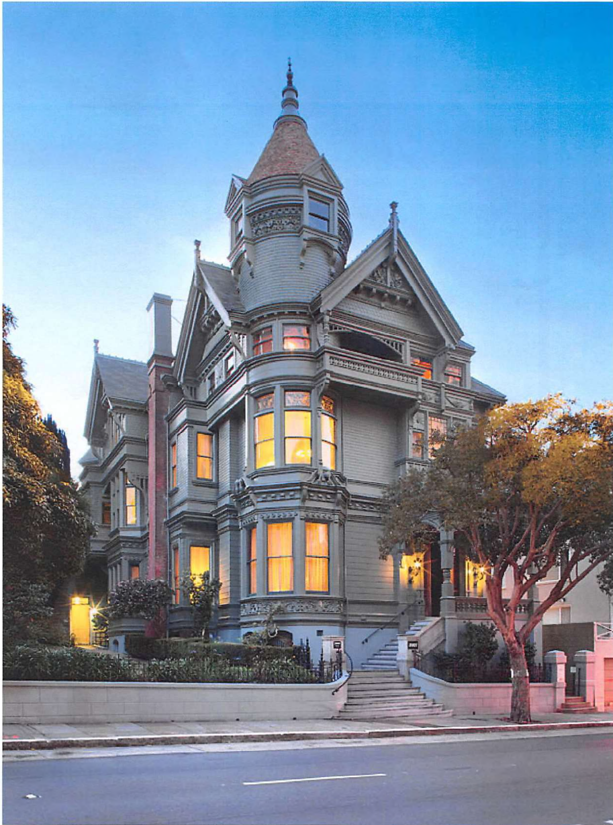
Teevan was selected to work on the repairs, restoration and repainting of the Haas-Lilienthal House, a 129-
