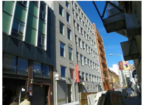
Stevenson Street facade, looking northwest. 103_3770.JPG. 3/1/2011
