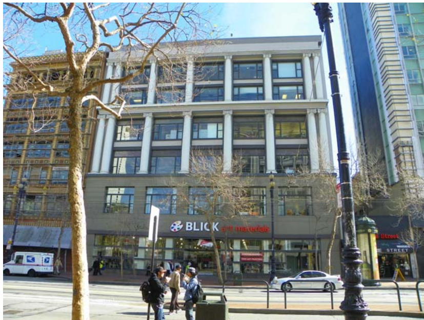
View of northwest facade. 103_3734.JPG 3/1/2011
