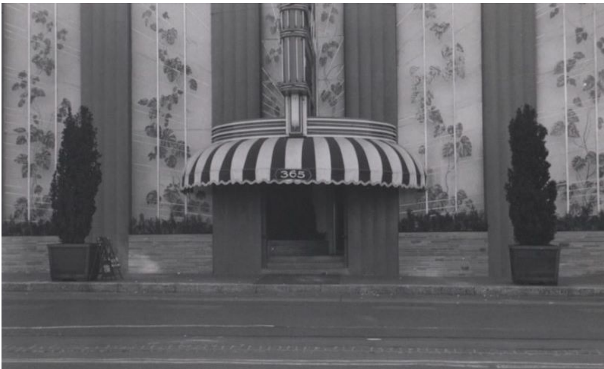
Front facade prior to addition of concrete block over stained glass and brick around entrance
