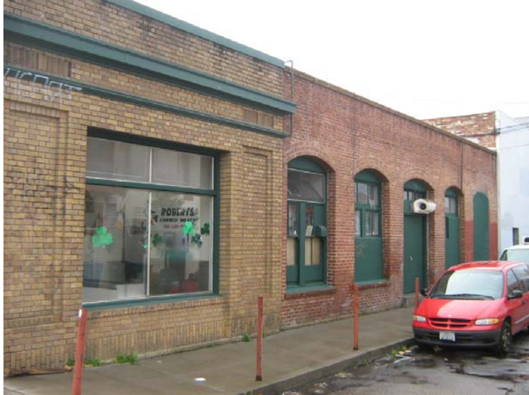
View of north façade. Source: Page and Turnbull
