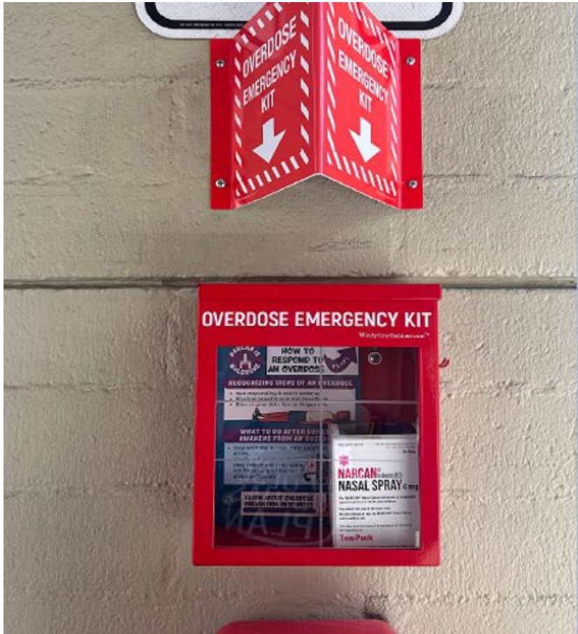
Overdose Emergency Kits being installed in many PSH sites, partnership with HSH and housing providers
