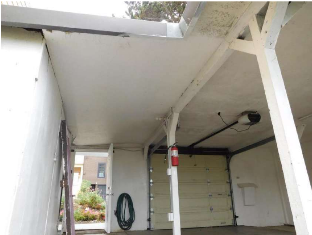
Figure 2: 617 Sanchez Street, front carport, interior
