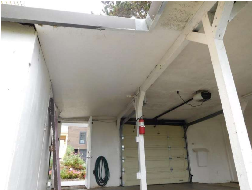
Figure 2: 617 Sanchez Street, front carport, interior
