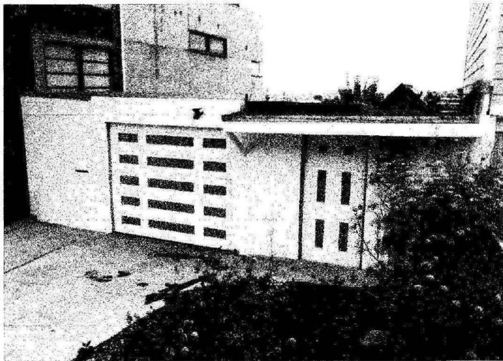
Figure 3. 617 Sanchez Street, garage structure. Source: 617 Sanchez Street HRE.
