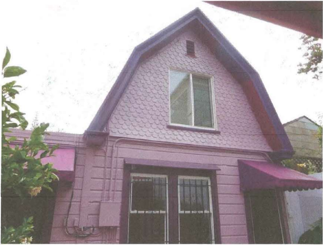
Figure 1. 617 Sanchez Street, residence building. Source: 617 Sanchez Street HRE.
