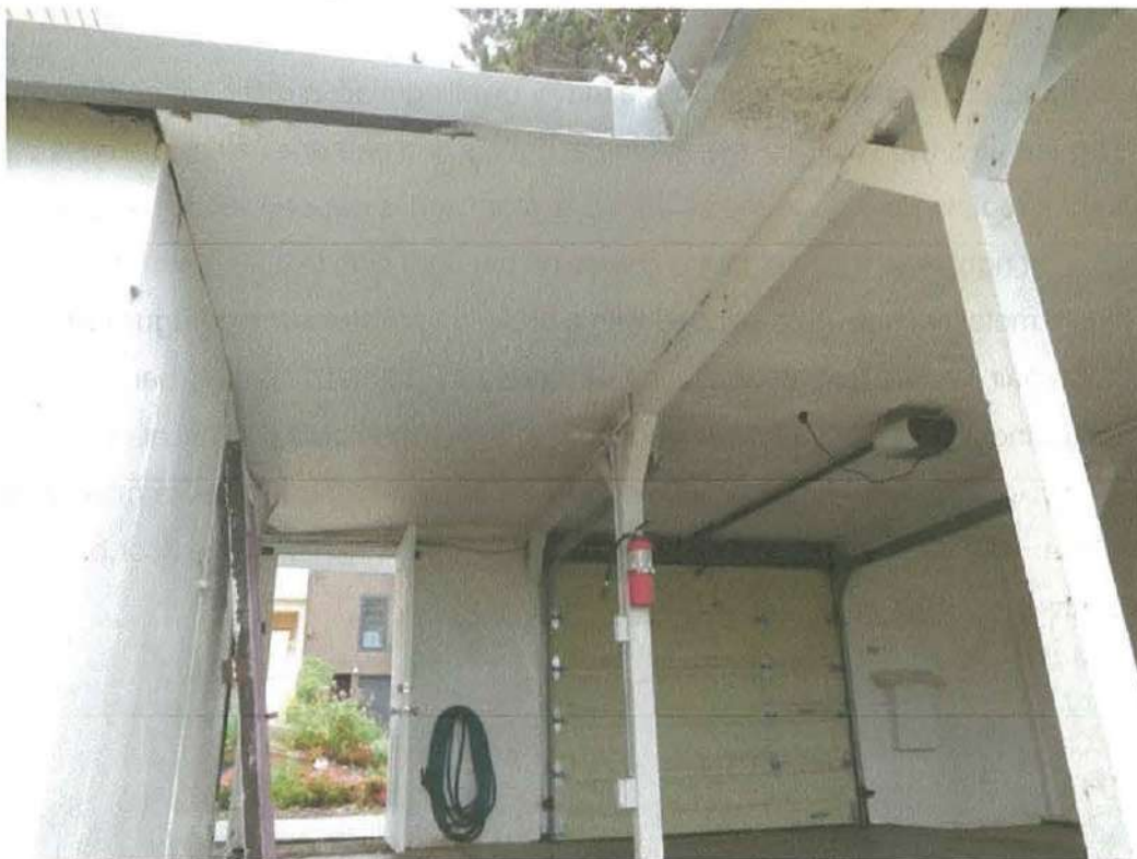
Figure 2: 617 Sanchez Street, front carport, interior
