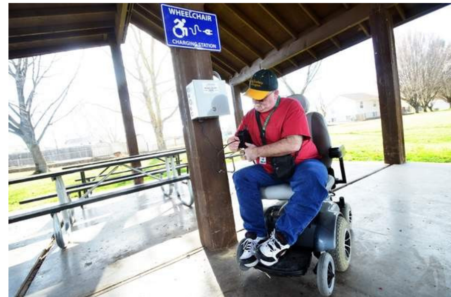
Image: Wheelchair charging station outdoors in a park and wheelchair user plugging in.
