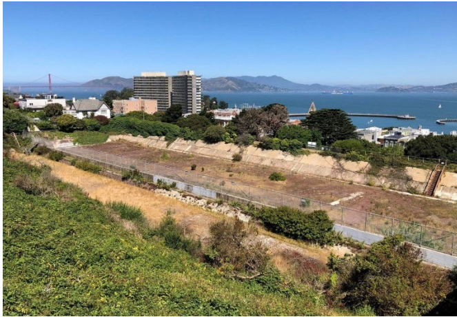
A view of the property before any work had started.
