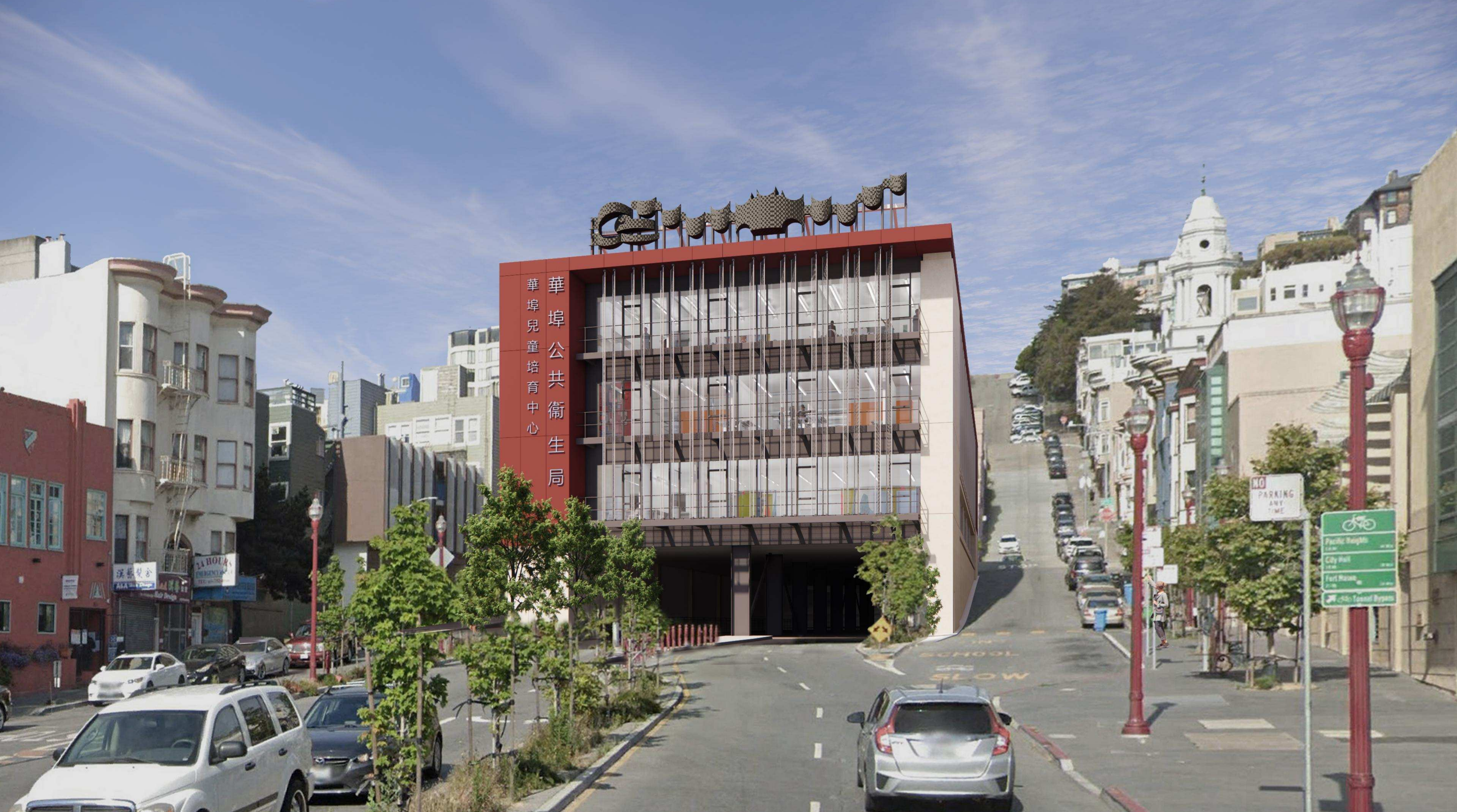
BROADWAY VIEW - ORIGINAL FINISH
