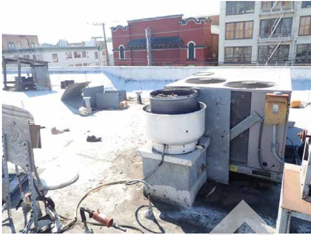
145. 2950-2978 16th St St roof
