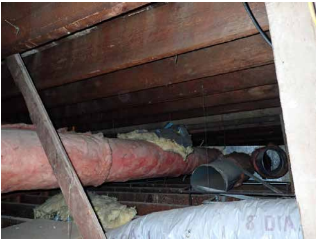
59. Wood framing Unit 2978
