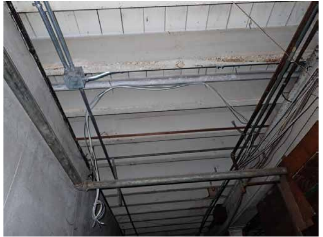
90. 1985 Mission St / 2950-2978 16th St framing
