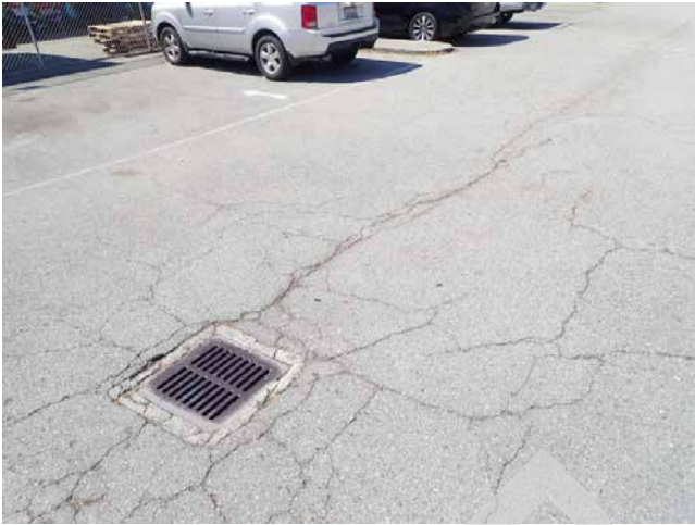
21. Typical parking lot storm drain
