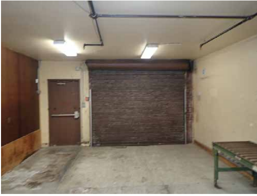
1979 Mission St- warehouse
