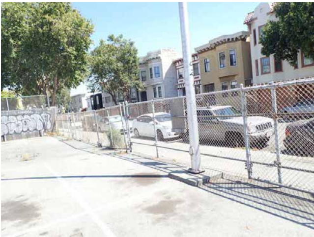
31. Parking lot chain link fence
