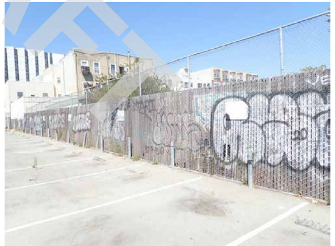
32. Parking lot chain link fence
