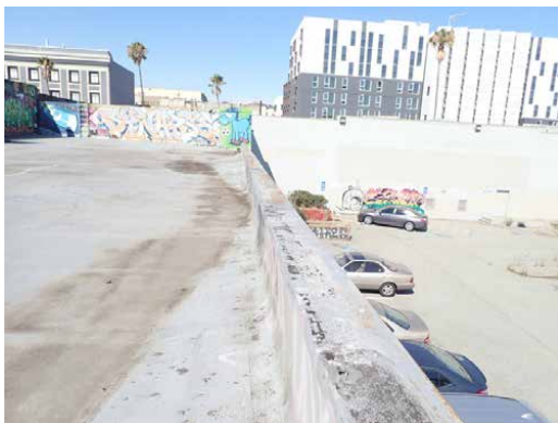
1985 Mission St modified bitumen cap sheet roof
