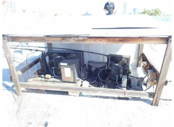
150. 2950-2978 16th St St roof
