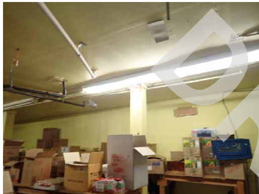
2970 16th St- basement storage area
