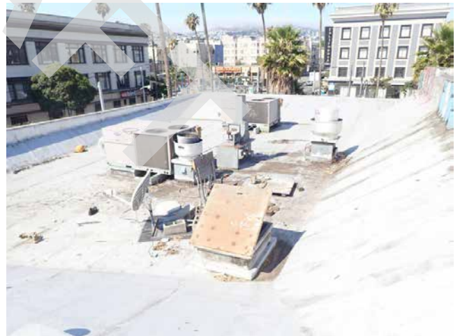
168. 2950-2978 16th St St roof
