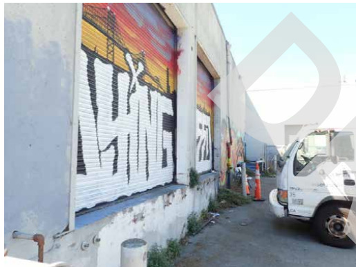
Loading dock area- 1985 Mission St
