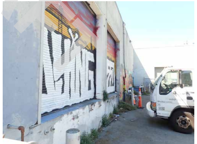
36. Loading dock area- 1985 Mission St
