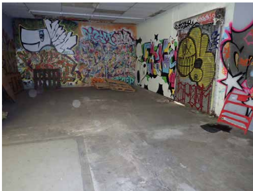
Concrete slab foundation in 1985 Mission St at loading dock area
