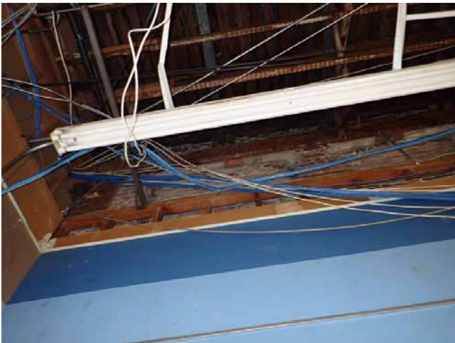
79. 1979 Mission St Framing
