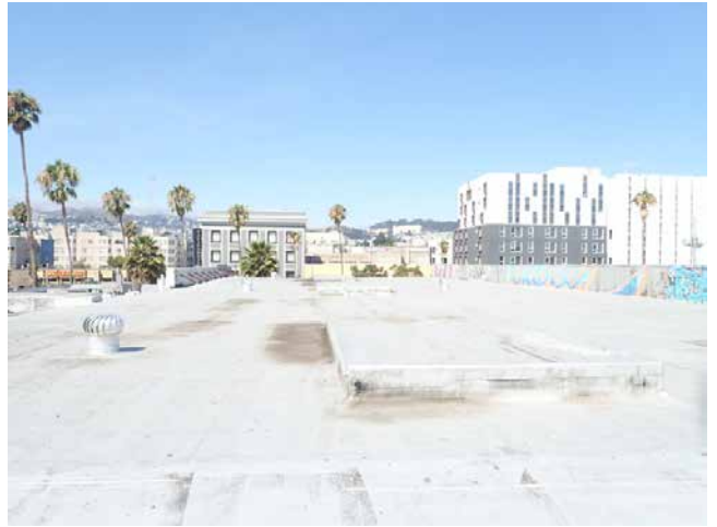
162. 2950-2978 16th St St roof
