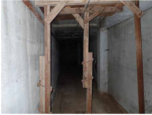
Wood shoring in basement area of 1985 Mission St / 2950-2978 16th St
