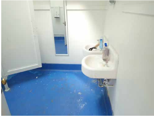
Unit 1985 mezzanine restroom
