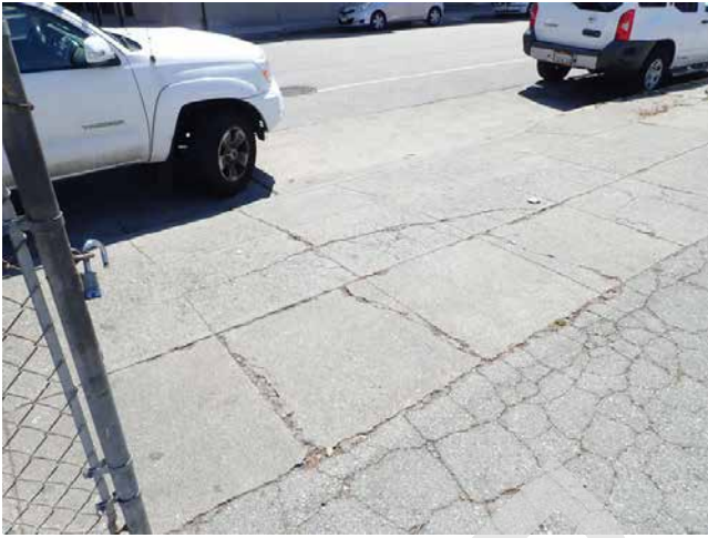
29. Cracked asphalt
