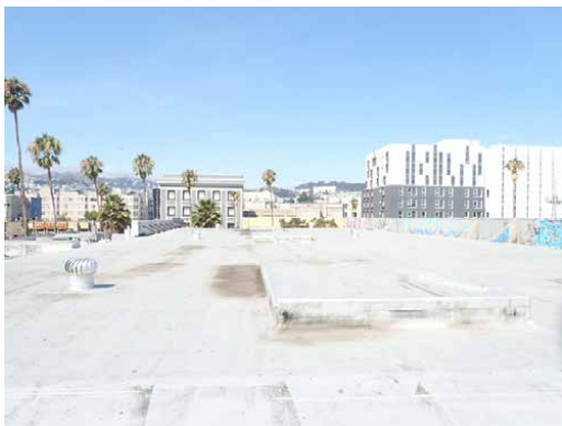
2950-2978 16th St St modified bitumen cap sheet roof
