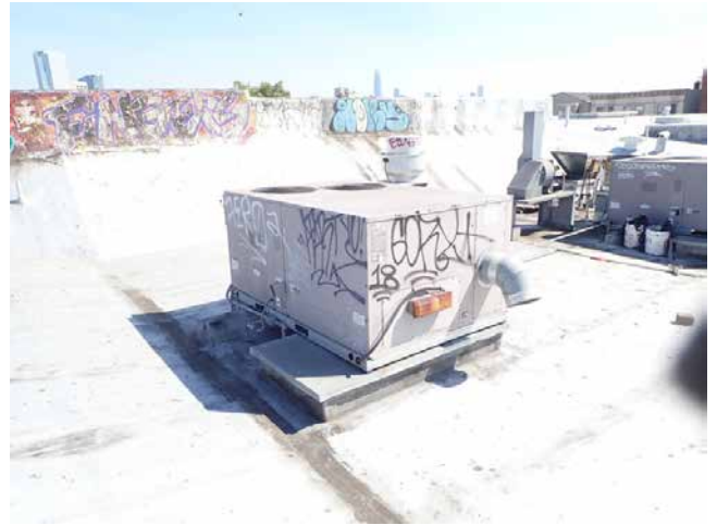
142. 2950-2978 16th St St roof
