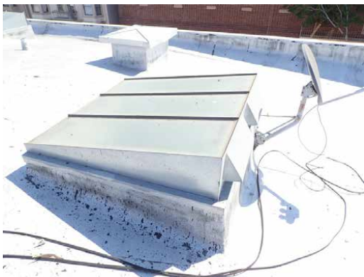
2950-2978 16th St St roof skylight
