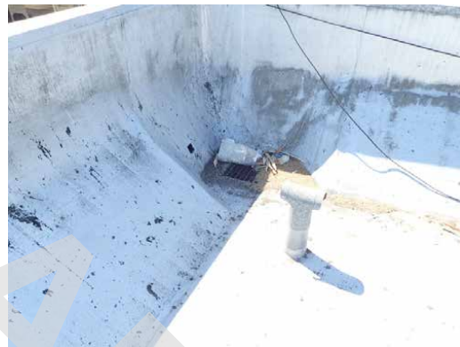
2950-2978 16th St St roof drain
