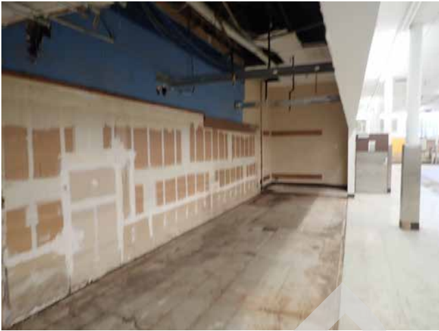
77. 1979 Mission St Framing
