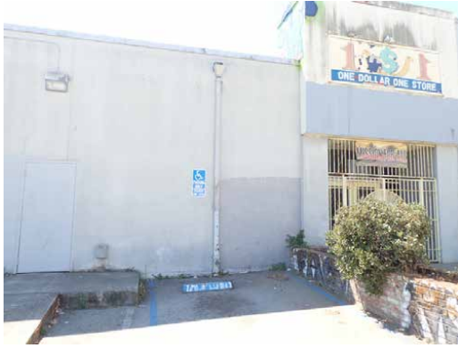
Typical roof downspout
