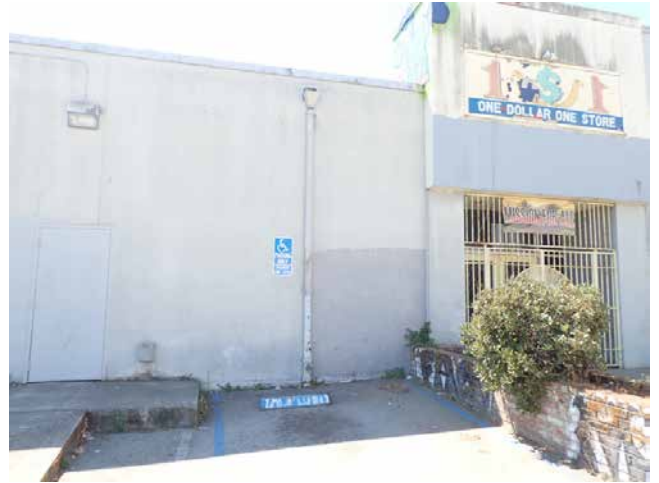
174. Typical roof downspout
