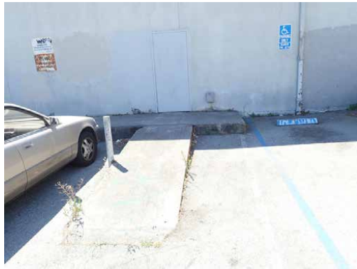
Warehouse area ramp 1985 Mission St.
