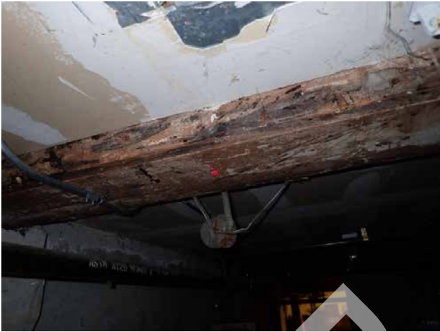
89. 1985 Mission St / 2950-2978 16th St framing
