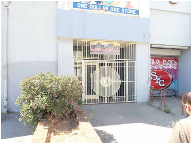
15. Sidewalk area to entrance to 1985 Mission St from Capp St.
