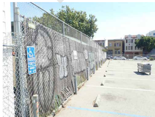
Parking lot chain link fence
