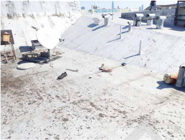
149. 2950-2978 16th St St roof
