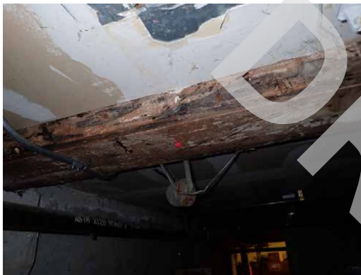
1985 Mission St / 2950-2978 16th St framing
