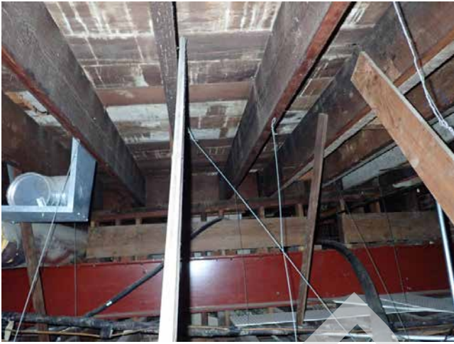
57. Steel and wood framing Unit 2978
