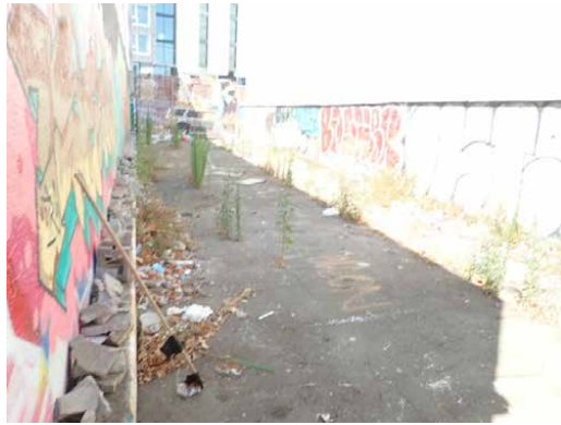
Gated driveway area- north-west side area along Mission
