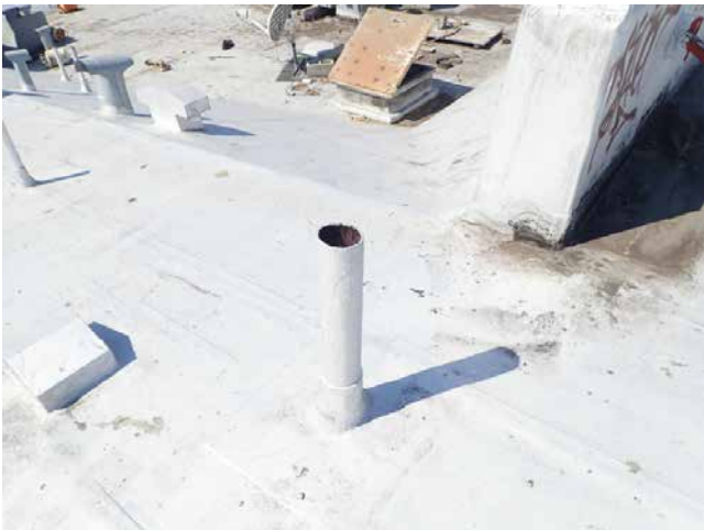
167. 2950-2978 16th St St roof
