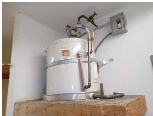
Typical electric water heater
