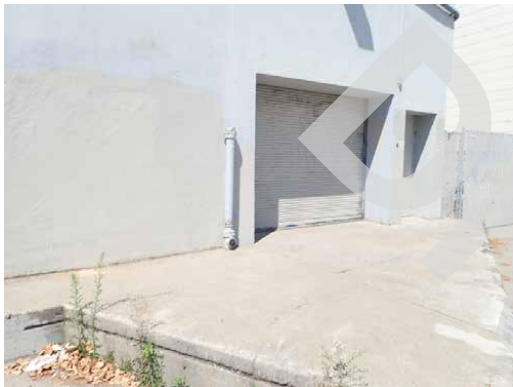
Disconnected downspout
