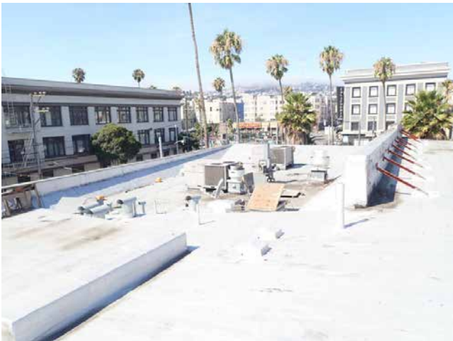
171. 2950-2978 16th St St roof
