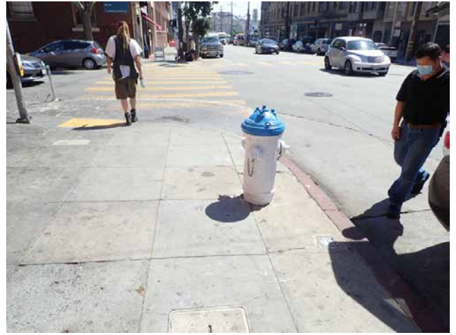
54. Street mounted fire hydrant
