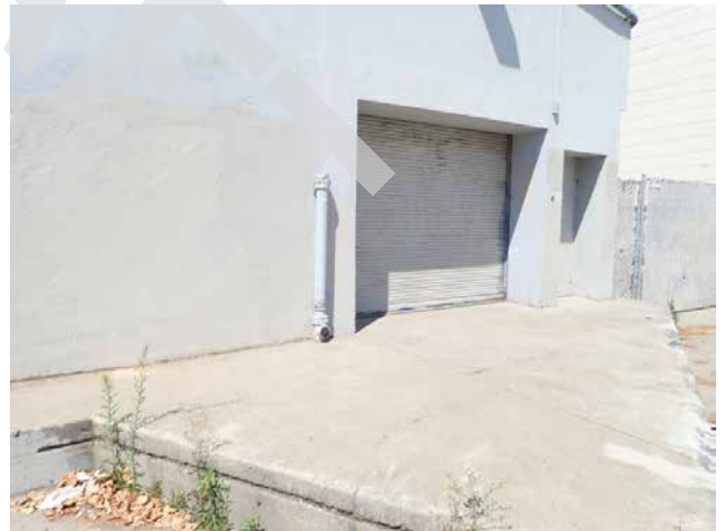
176. Disconnected downspout
