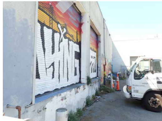
Loading dock area- 1985 Mission St
