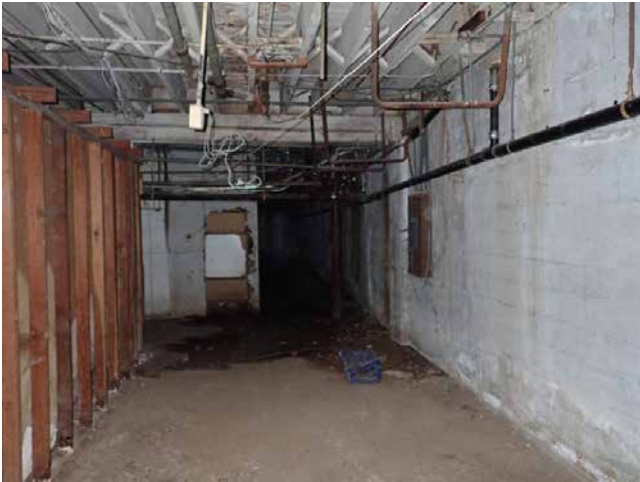
55. Basement Area-concrete slab foundation with concrete sidewalls
