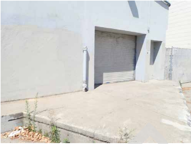
37. Loading dock area- 1979 Mission St
