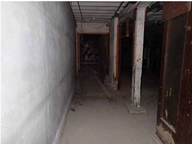
91. 1985 Mission St / 2950-2978 16th St framing
