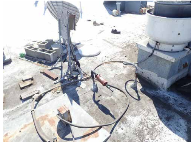
146. 2950-2978 16th St St roof
