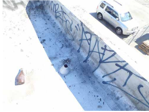
1985 Mission St roof parapet
