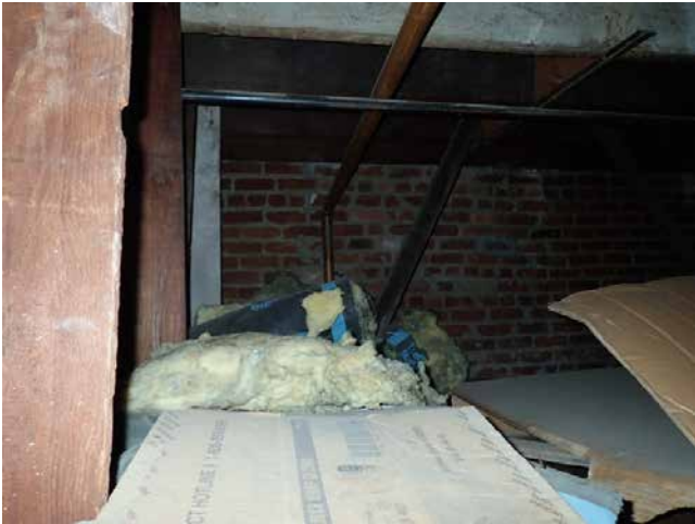
83. 1985 Mission St / 2950-2978 16th St framing
