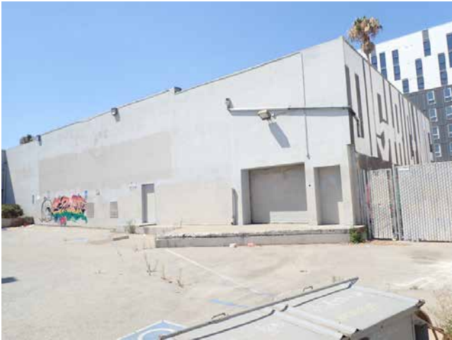
39. Loading dock area- 1979 Mission St
