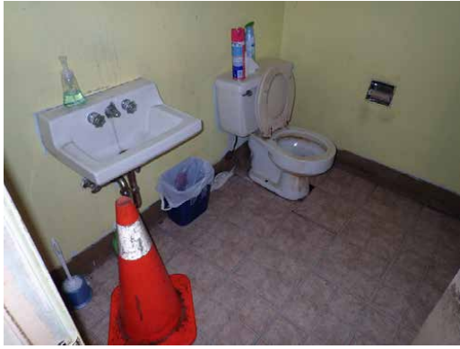
Unit 2970 mezzanine restroom
