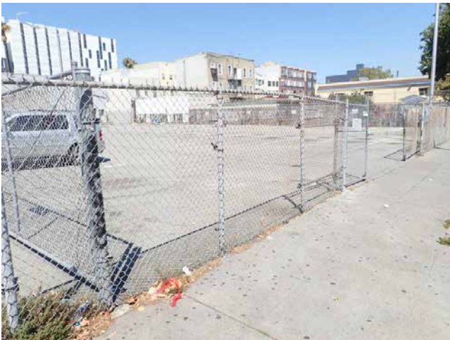
47. Parking lot security gate
