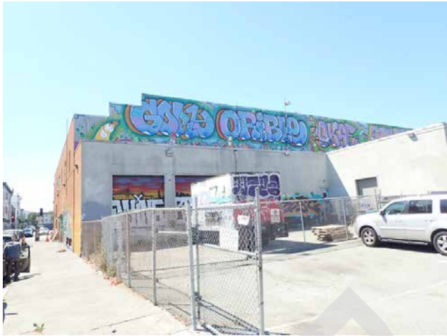
33. Gate to parking lot
