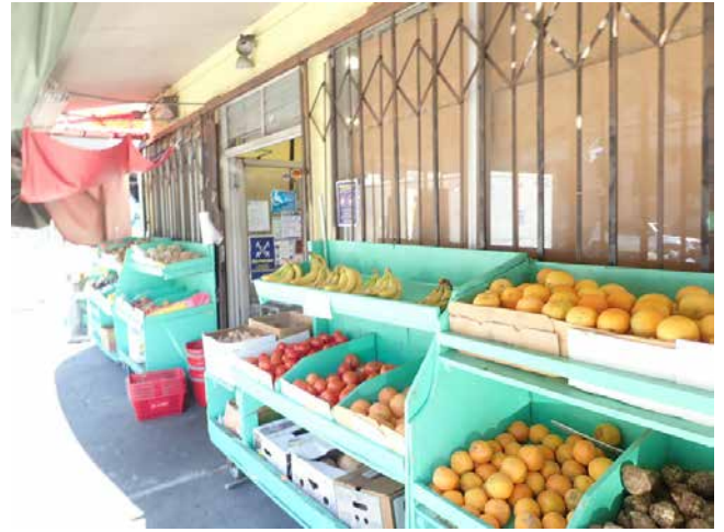
66. Storefront windows and doors- 2970-2972 16th St.
