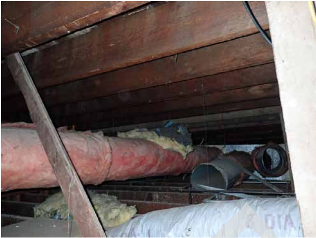
85. 1985 Mission St / 2950-2978 16th St framing
