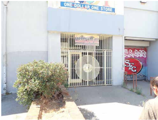
Landscaped area at east side entrance to 1985 Mission St Sidewalk area to entrance to 1985 Mission St from Capp St.
