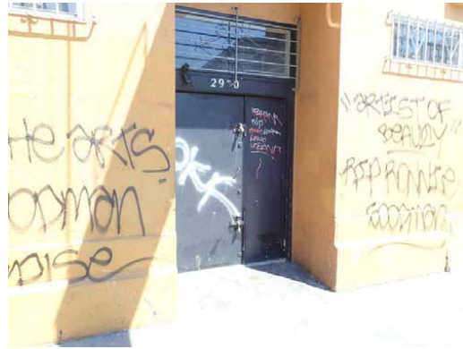
2950 16th St entrance door
