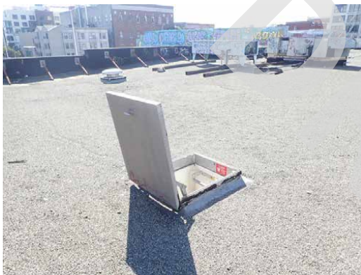
1979 Mission St roof hatch
