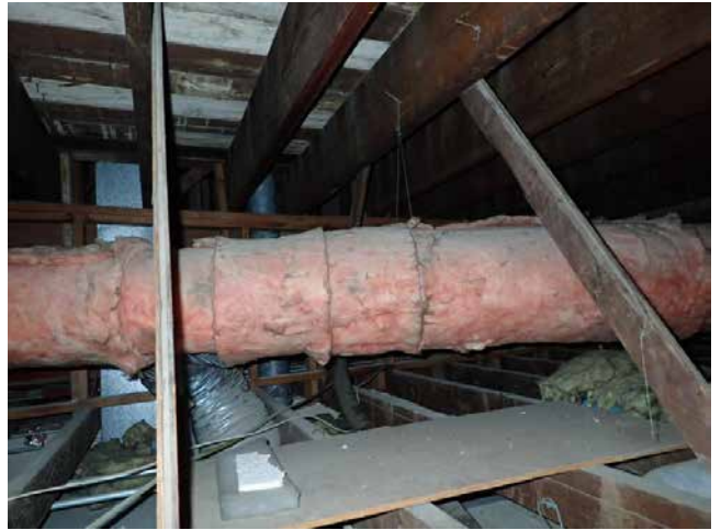
86. 1985 Mission St / 2950-2978 16th St framing
