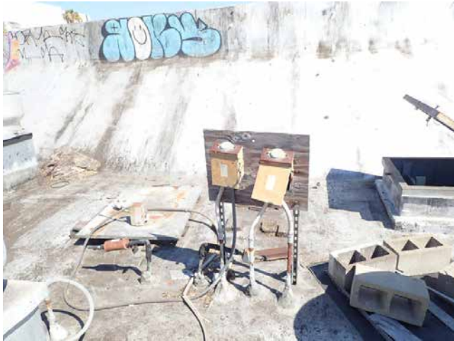
147. 2950-2978 16th St St roof
