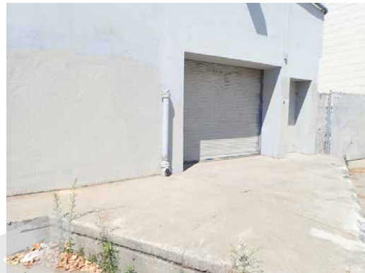
Loading dock area- 1979 Mission St
