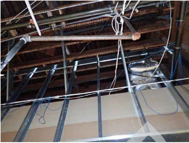
81. 1979 Mission St Framing
