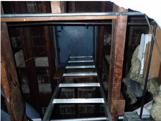
87. 1985 Mission St / 2950-2978 16th St framing
