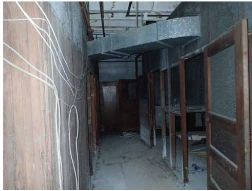
Unit 1985- basement area
