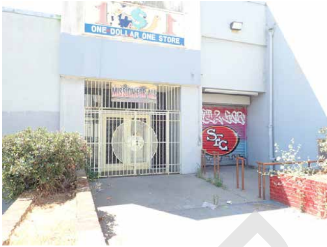
65. Landscape planters at entrance to 1885 Mission St.
