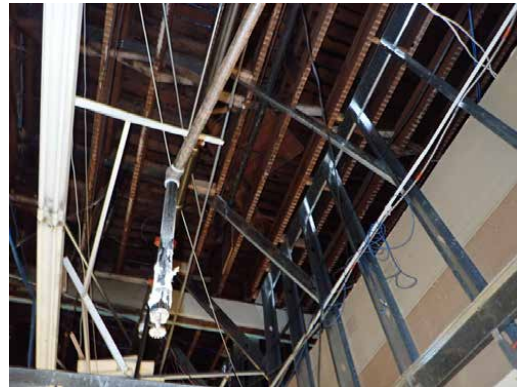
1979 Mission St wood roof Framing
