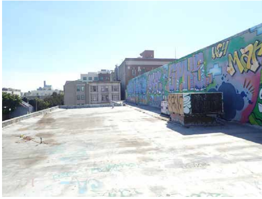
1985 Mission St modified bitumen cap sheet roof
