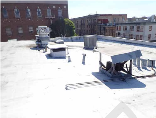
169. 2950-2978 16th St St roof
