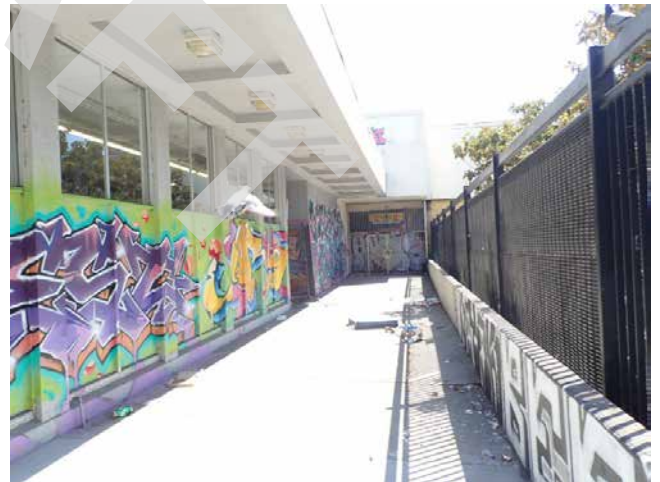
16. Sidewalk area to entrance to 1985 Mission St along Mission St.
