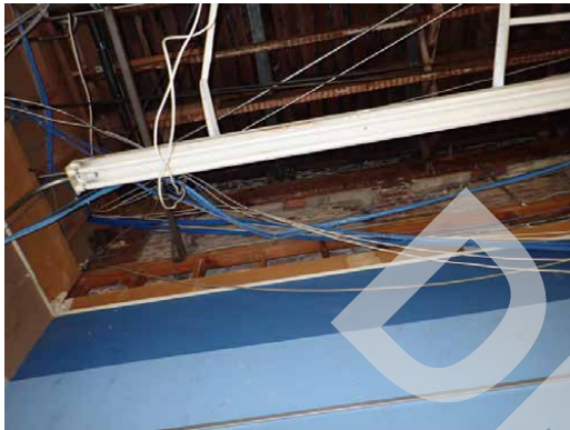
1979 Mission St Framing
