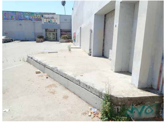
38. Loading dock area- 1979 Mission St
