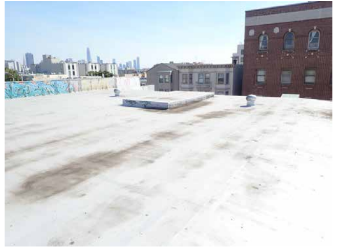
170. 2950-2978 16th St St roof
