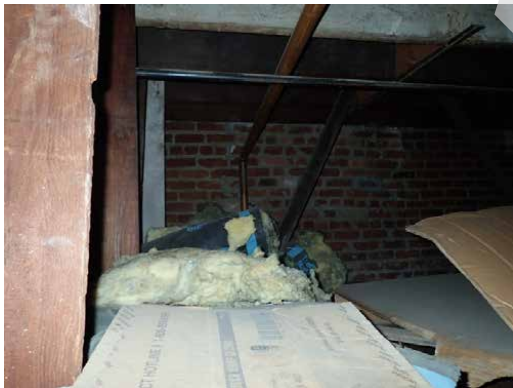
1985 Mission St / 2950-2978 16th St wood and brick framing
