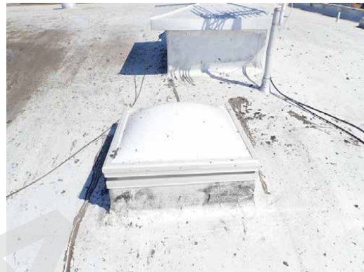
2950-2978 16th St St roof skylight
