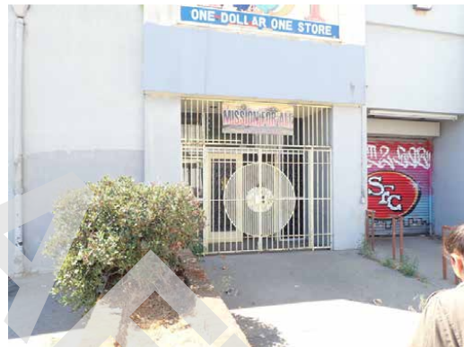
Sidewalk area to entrance to 1985 Mission St from Capp St.
