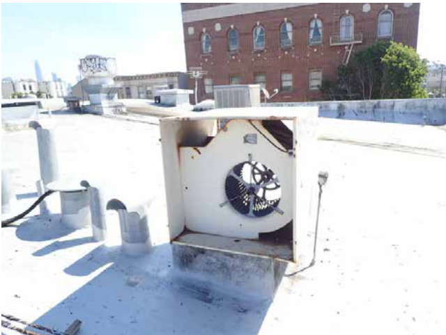
151. 2950-2978 16th St St roof
