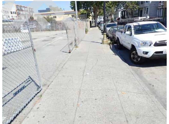
44. Parking lot entrance apron
