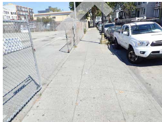
Parking lot entrance apron
