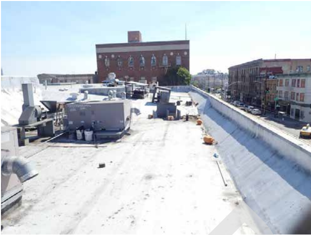
141. 2950-2978 16th St St roof
