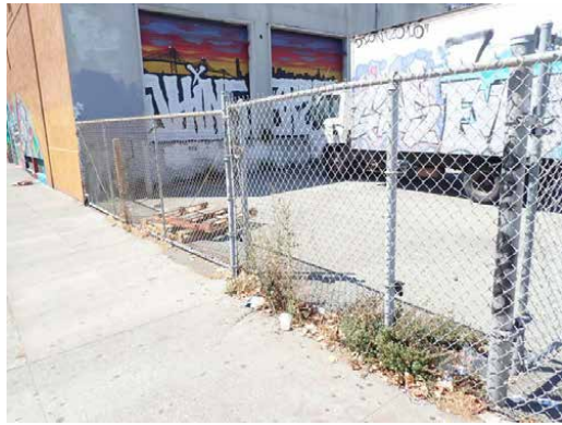
Parking lot chain link fence
