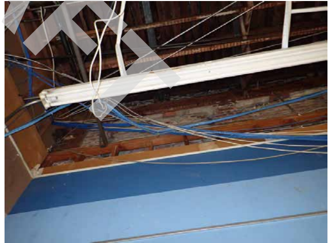
56. Brick and wood framing Unit 2978
