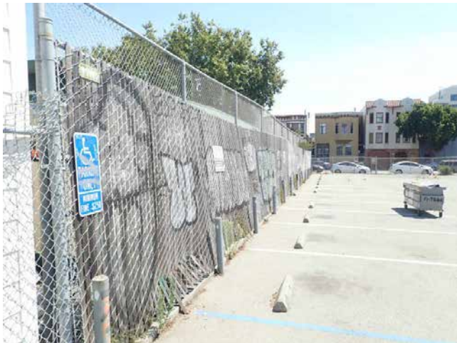
35. Parking lot chain link fence
