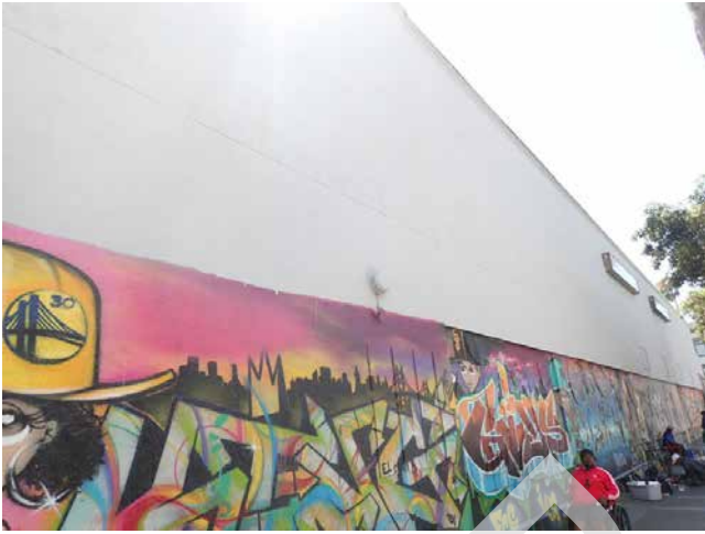
61. Fire alarm bell for 1979 Mission St
