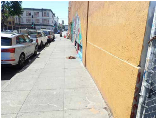
Public sidewalk area- east elevation along Capp St
