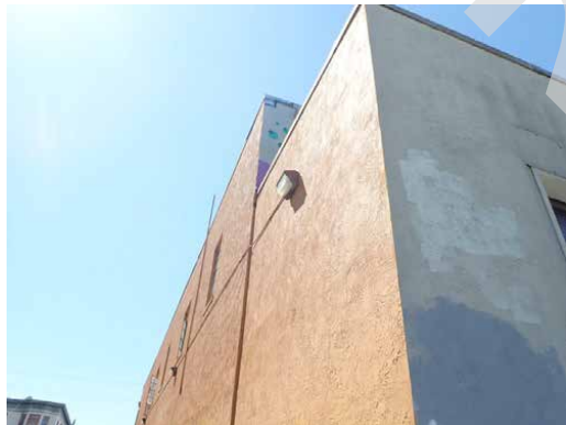
Typical stucco of brick
