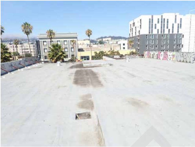
165. 2950-2978 16th St St roof
