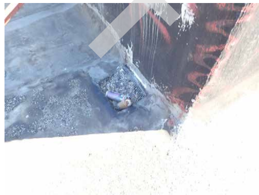
1985 Mission St roof drain
