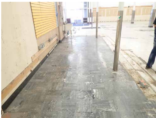
Concrete slab foundation in 1979 Mission St.
