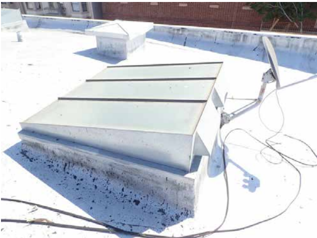
159. 2950-2978 16th St St roof
