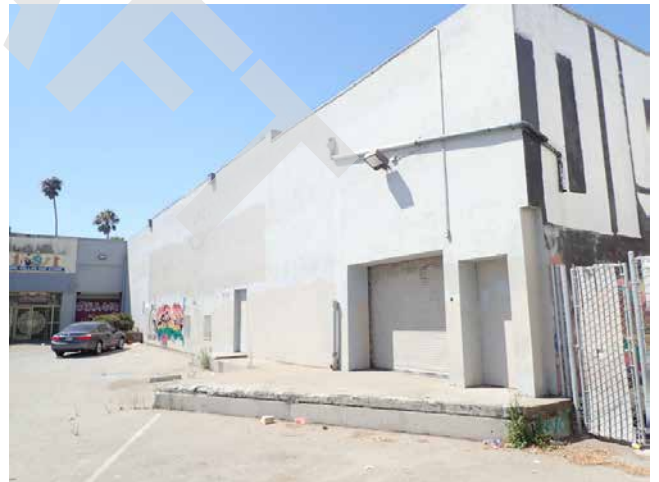
172. Roof downspout modification
