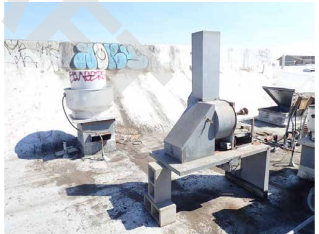
144. 2950-2978 16th St St roof
