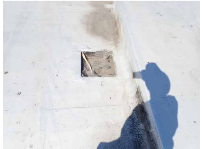
166. 2950-2978 16th St St roof
