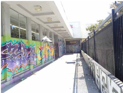
Sidewalk area to entrance to 1985 Mission St along Mission St.
