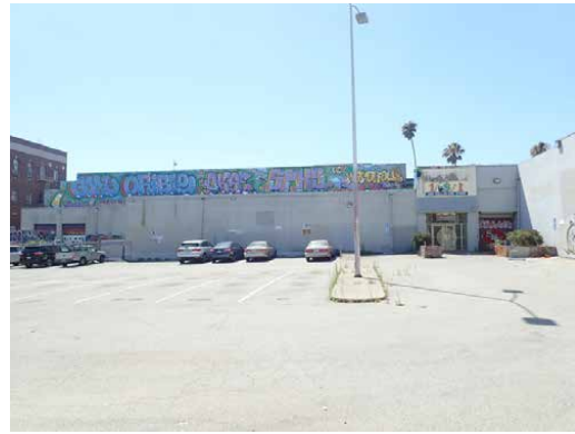
Typical parking lot pole mounted lighting
