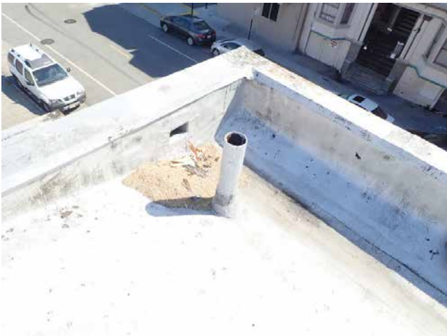
163. 2950-2978 16th St St roof
