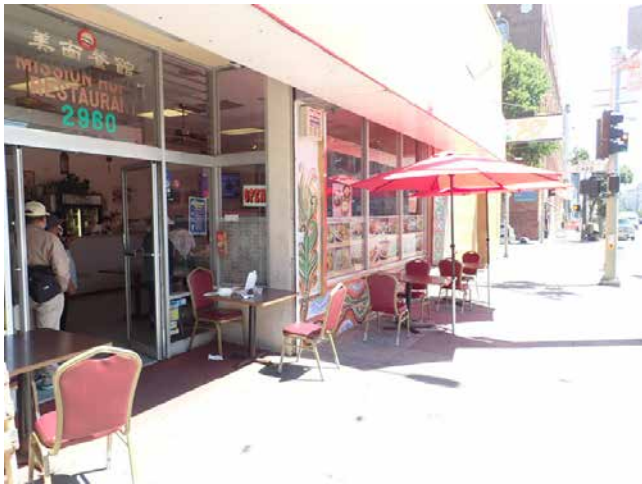
67. Typical store front windows and doors- 2960 16th St.
