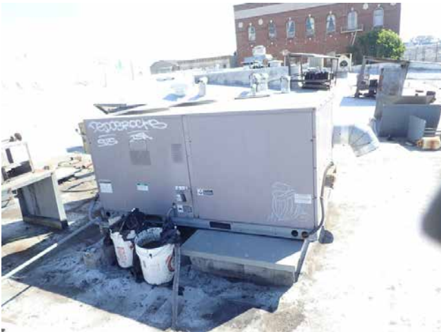
143. 2950-2978 16th St St roof
