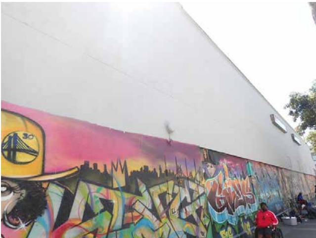
203. 1979 Mission St- fire alarm bell
