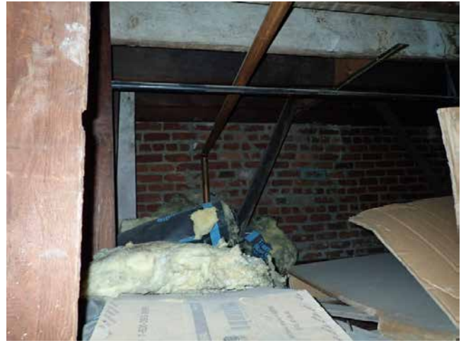
58. Brick and wood framing Unit 2978
