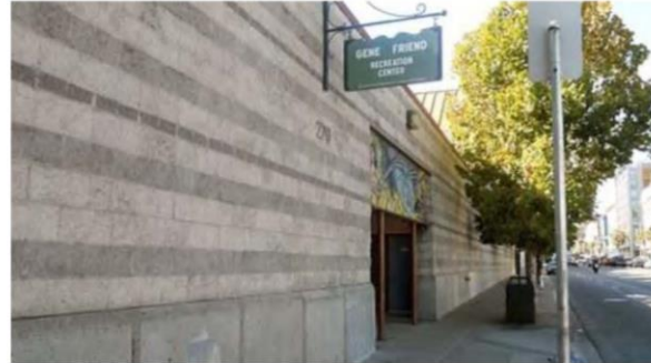
EXISTING - 6 TH STREET ENTRANCE
