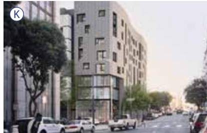
555 Larkin Street/ 500 Turk Street
