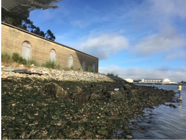
East side of Torpedo Storehouse site, looking north.
