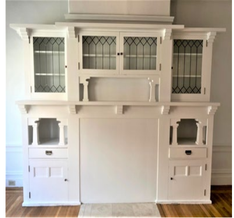
Figure 2: Built-in Cabinets Figura 2: Gabinetes empotrados
