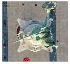
Image 2: Detail of bio-growth and general soiling on the bronze figure.
