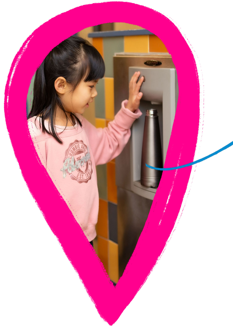
Water bottle filling station at school
