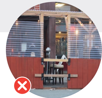
This is a non-compliant gap because of the overhead and pathway obstructions.
