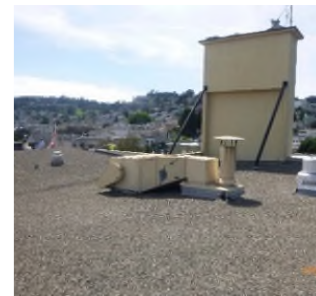
Fire Station Hose Tower
