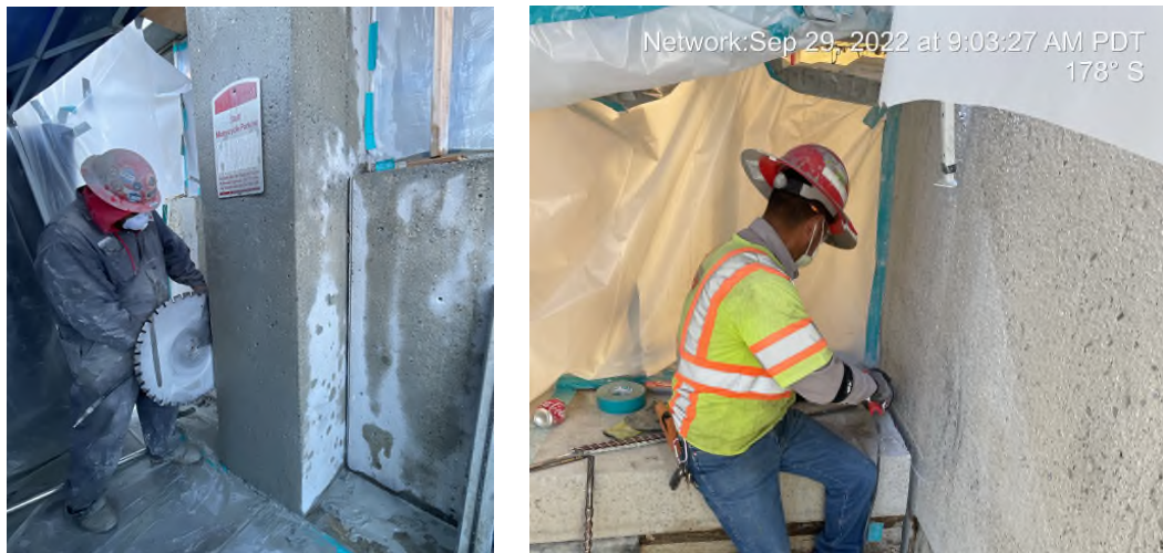
Exterior sawcutting at spandrel locations
