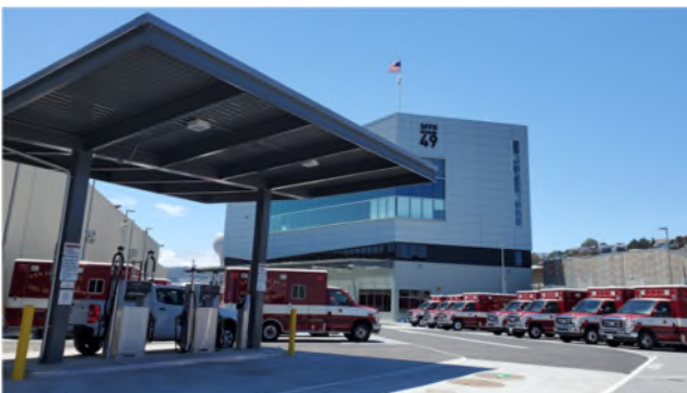
Constructed new Ambulance Deployment Facility (New SFFD Station 49)
