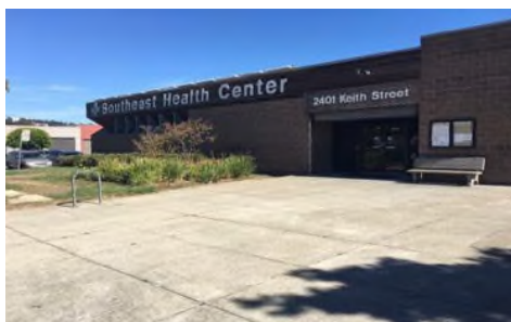
Existing SE Health Center
