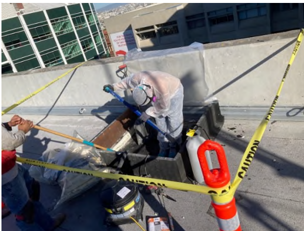
Roof Abatement and Demolition
