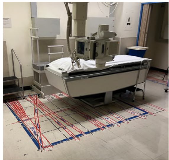
Radiology Rooms 1X65 and 1X61 Rebar and Post Tension (PT) Floor Scanning and Layout
