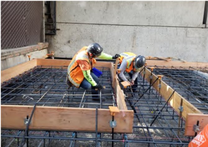
New Mechanical Concrete Pads for new Chillers
