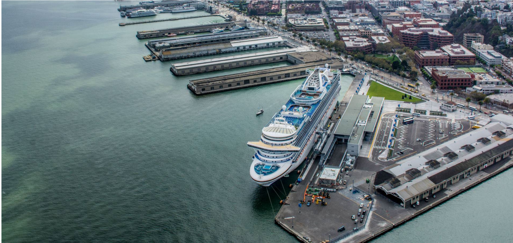
Pier 27 Cruise Terminal
