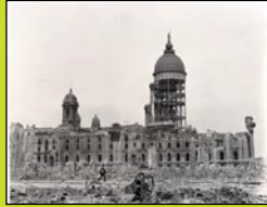
1906, City Hall after earthquake
