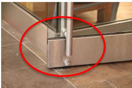
*Example of lower kick plate blocked by lock and door hardware.*
