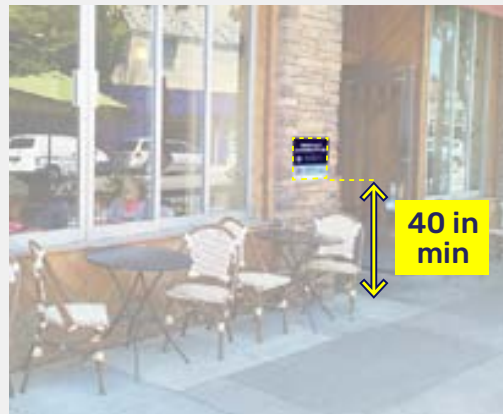
Sidewalk Signage on building face, mounted onto opaque wall.
