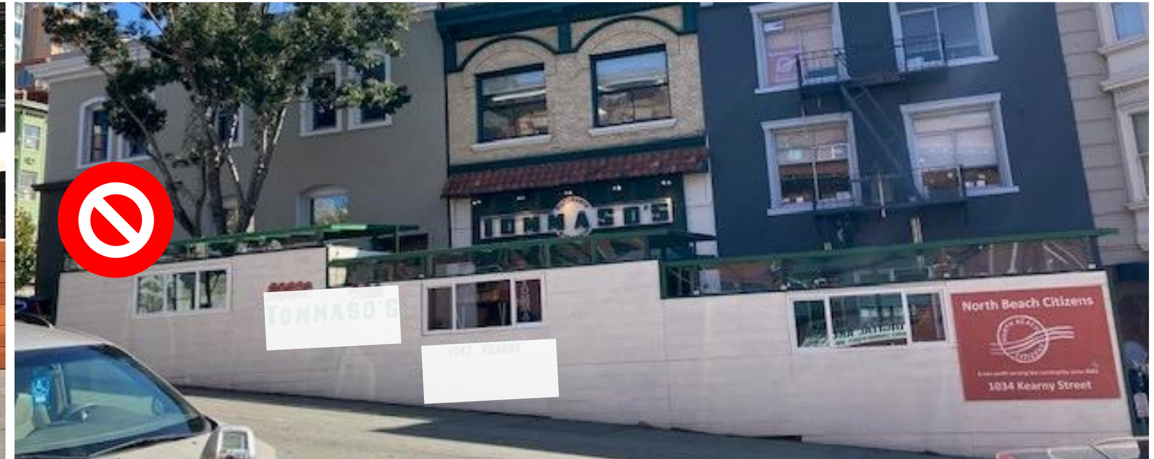
Blocking multiple building ingress and egress points
