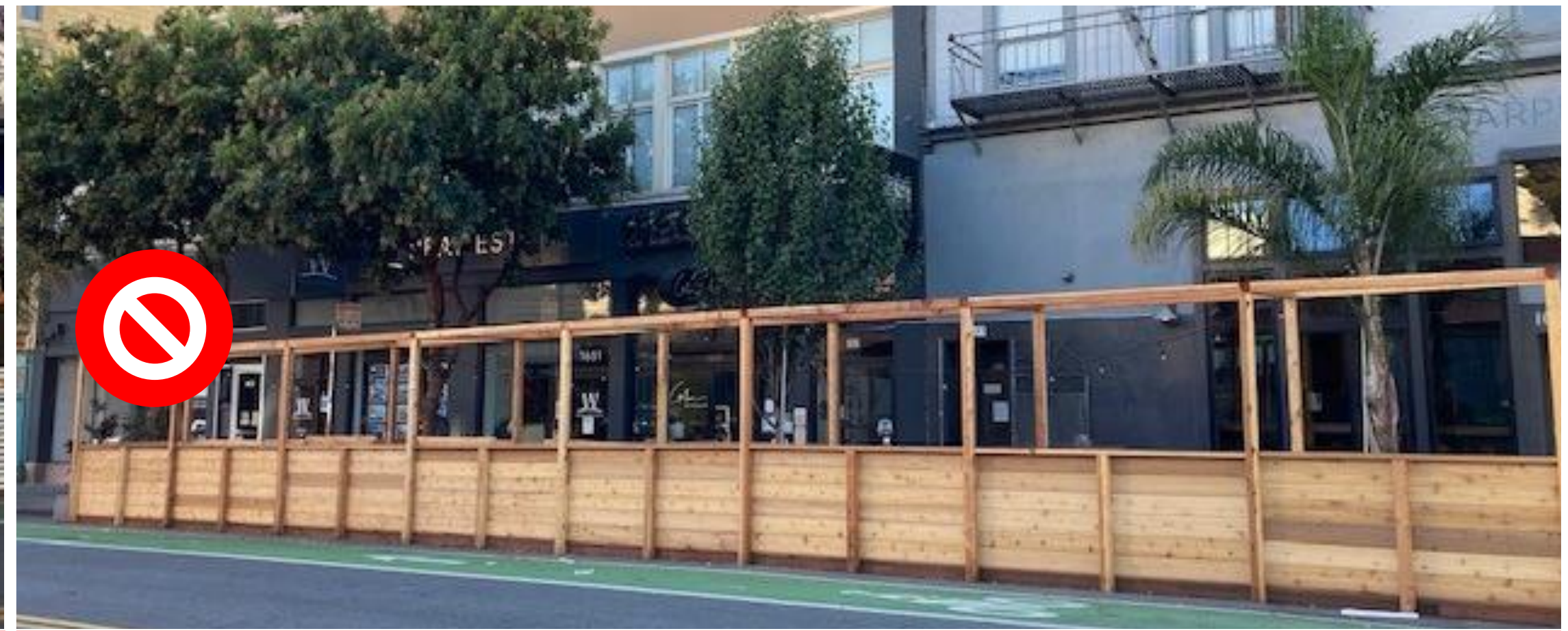
No through-access for firefighting ladders and medical gurneys
