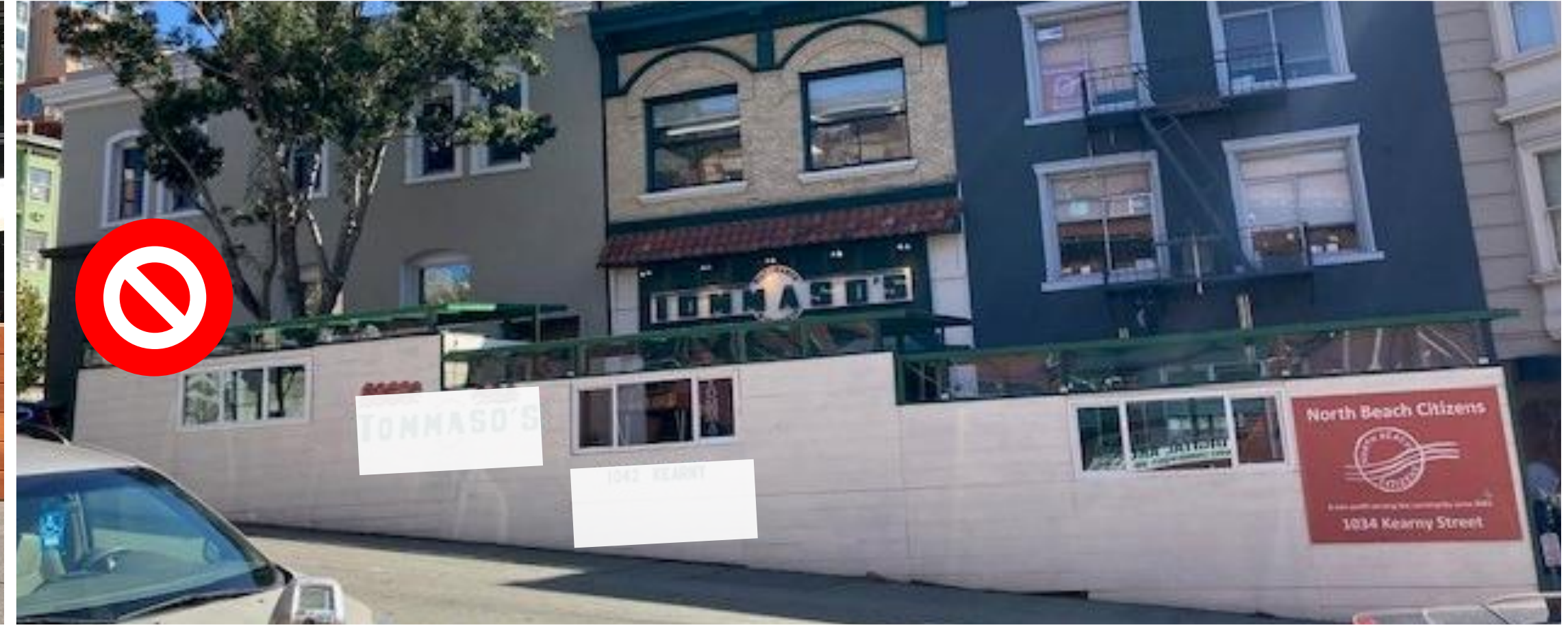
Blocking multiple building ingress and egress points
