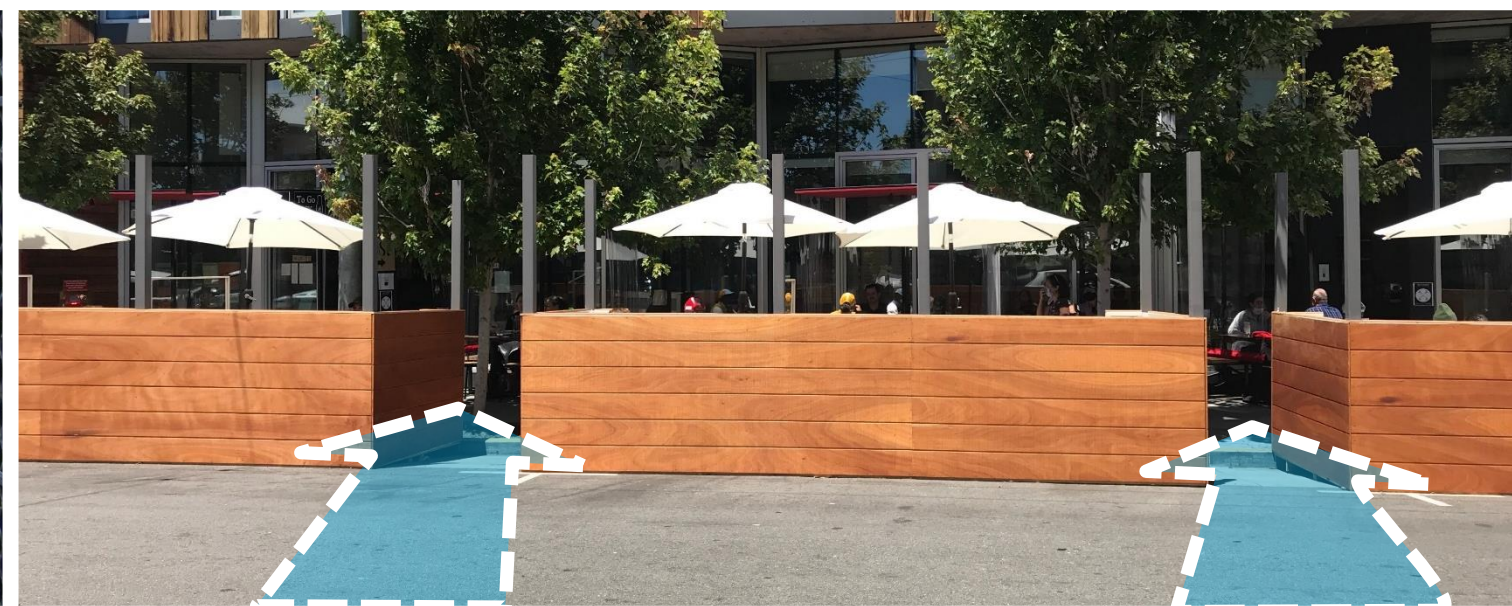
3-foot Access Gaps, Open to the Sky
