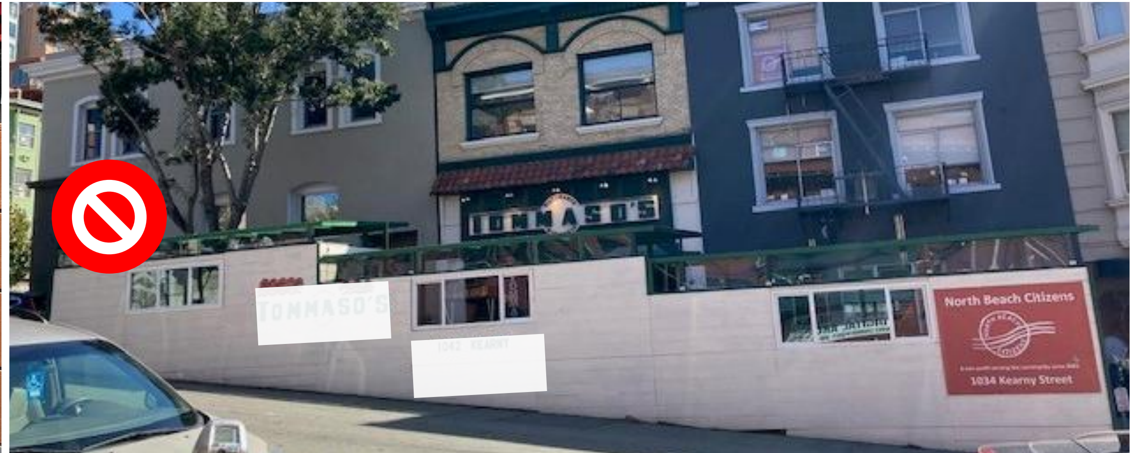
Blocking multiple building ingress and egress points
