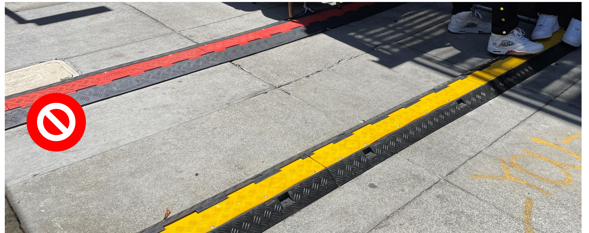
Cable ramps are bad for wheelchairs
