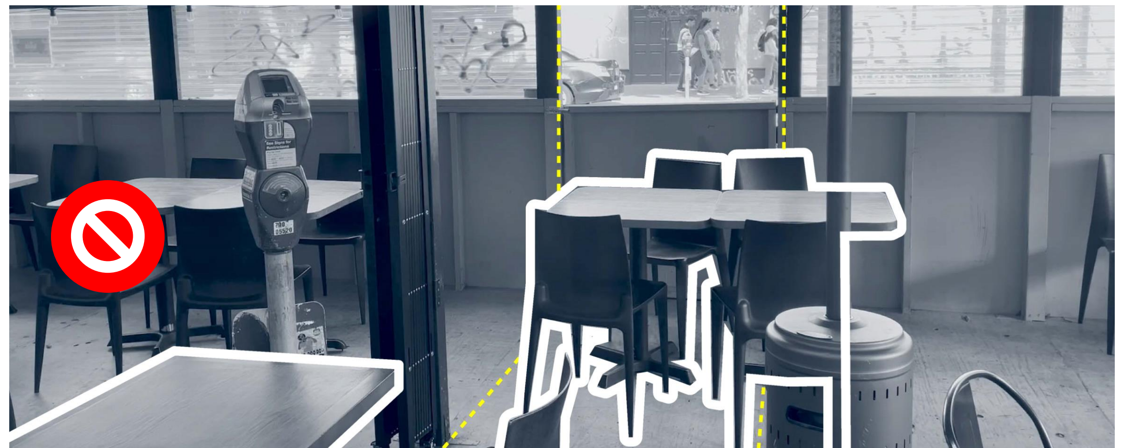
Solid wall in 3' gap, tables & chairs in path of travel
