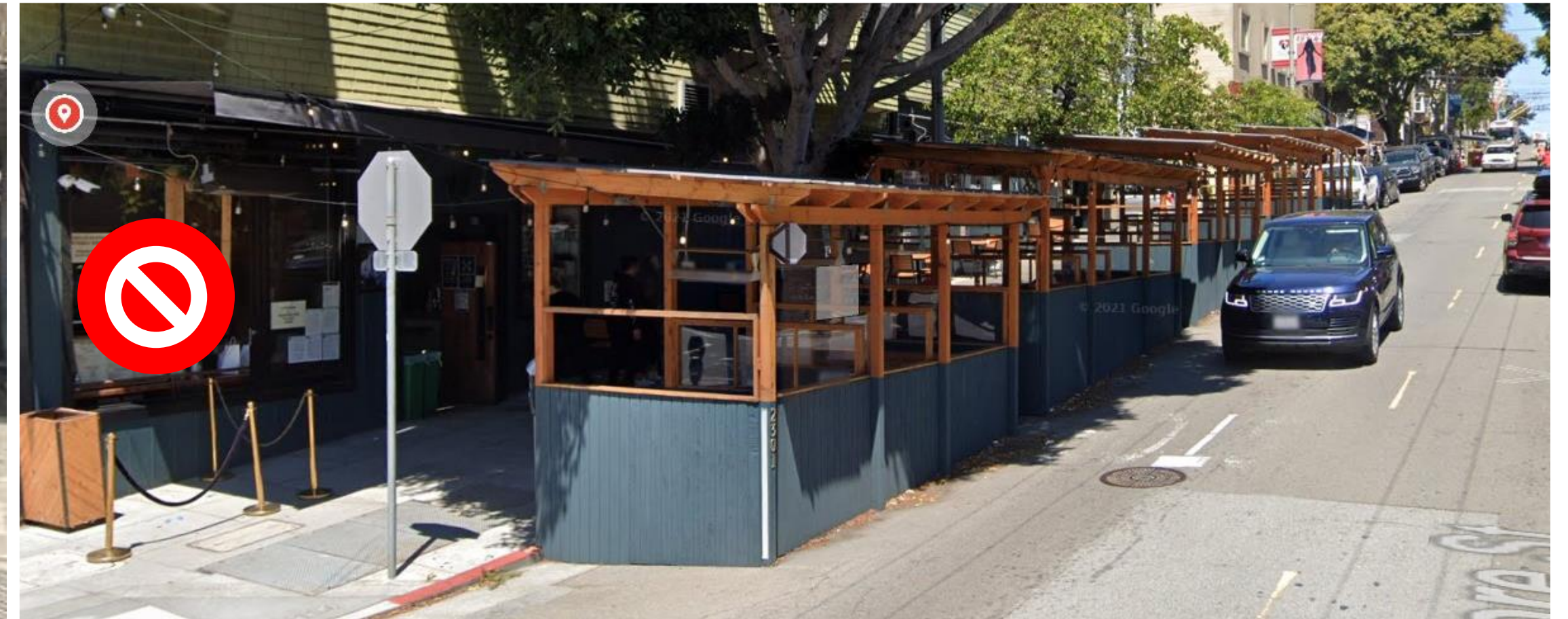
Difficult for pedestrians to see oncoming cars
