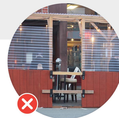
This is a non-compliant gap because of the overhead and pathway obstructions.
