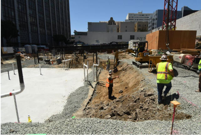
Construction underway at 500 Turk
