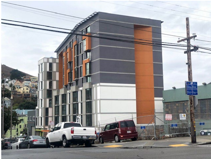
Casa Adelante - 1296 Shotwell construction complete and fully-occupied
