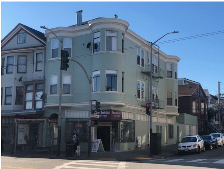
3800 Mission Street – completed June 2019
