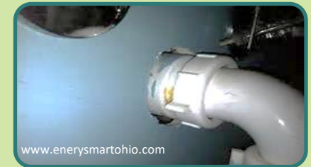
Openings and gaps where wires, conduits, pipes, sillcocks, ducts come into the building from the exterior through the walls, ceilings, floors, the backs of cabinets into the apartment unit
