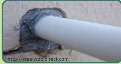
Steel wool reinforced with sealer
