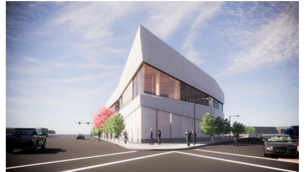
Carpenter's Union Hall establishing view over 3rd Street and Cargo Street, rendering by Mithun and lightly edited by YIMBY
