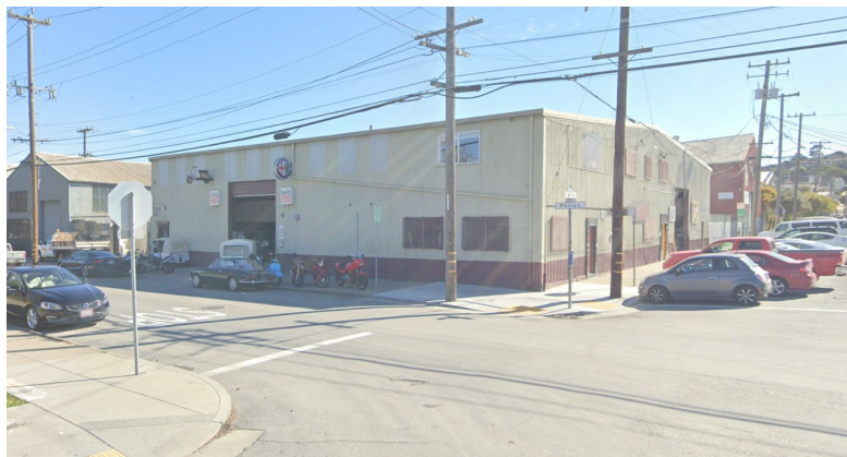
C East Corner of Phelps-Jerrold Intersection
