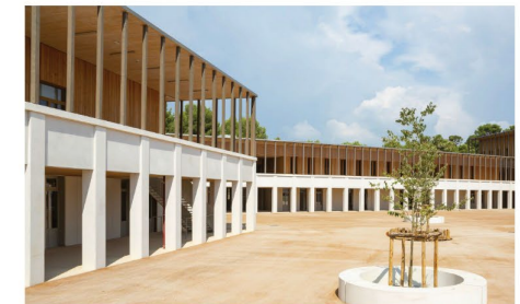
COLONNADES ON TWO FLOORS
