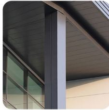
6 PAINTED STEEL COLUMNS
