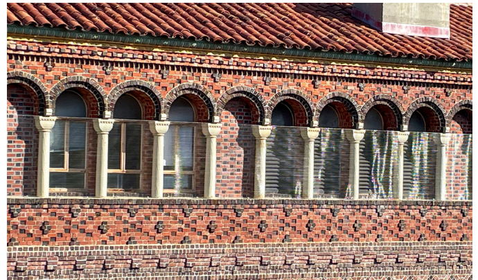
Protective Netting Installed on Historic Buildings
