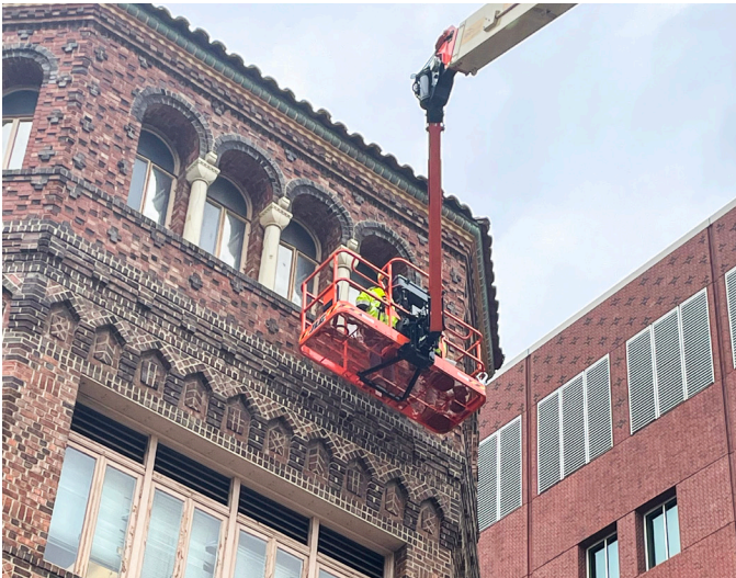
Routine Maintenance of Historic Campus Buildings
