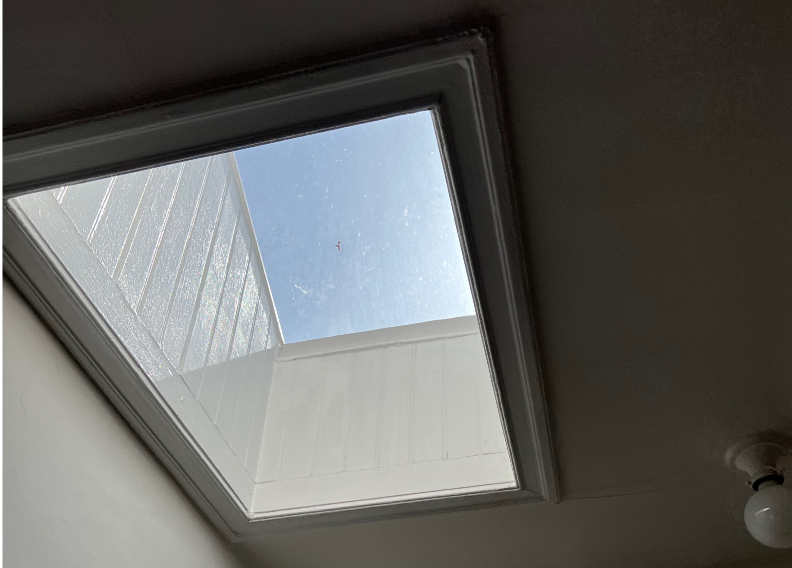
Photo 6 553 Wisconsin Street Skylight
