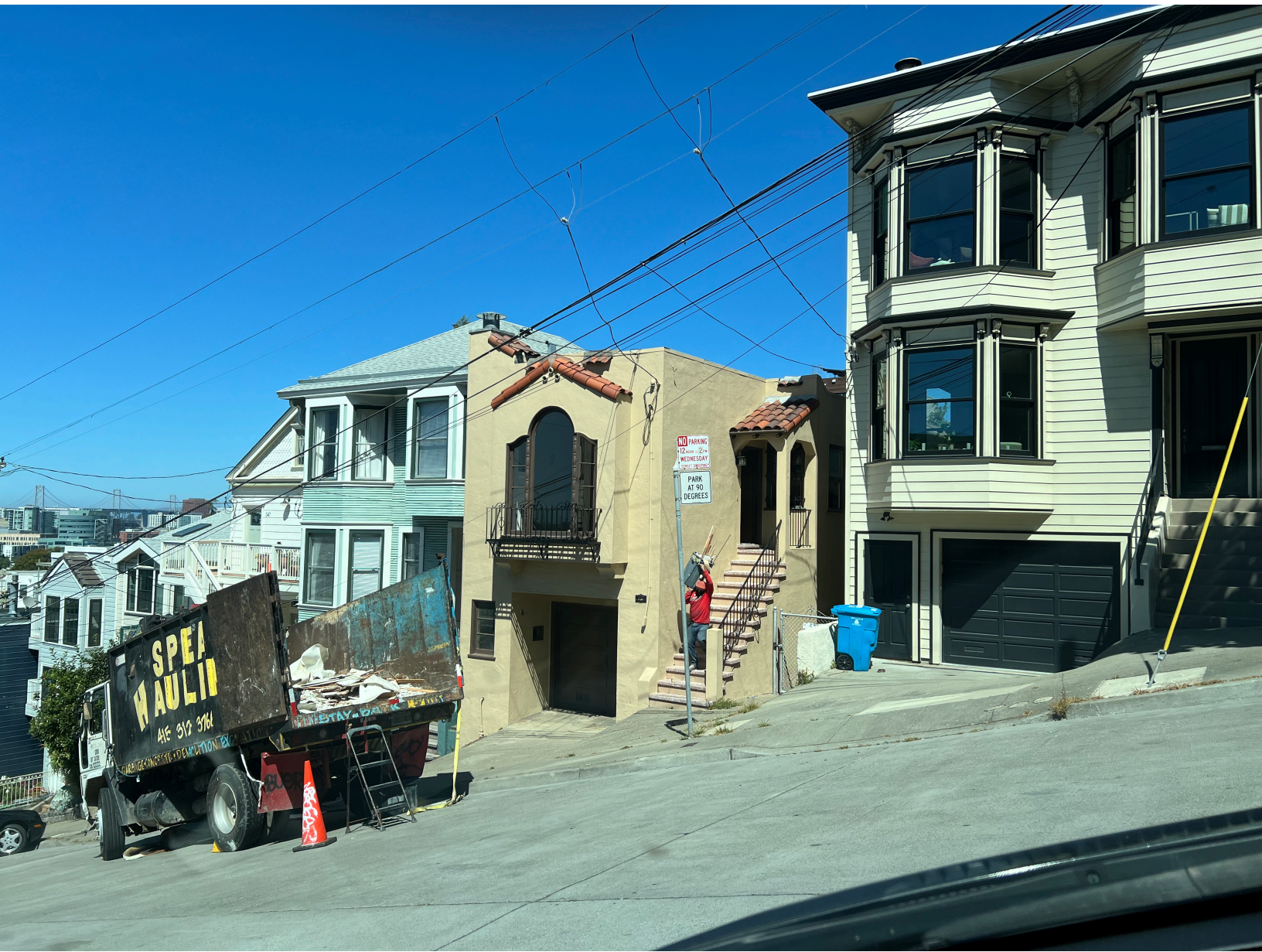
Photo 1 Loading lath and plaster at 557 Wisconsin Street
