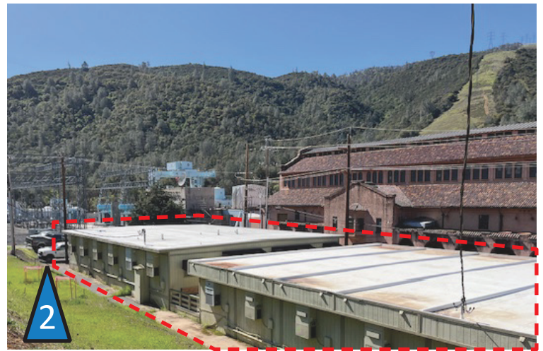
EXISTING 1-STORY MODULARS
