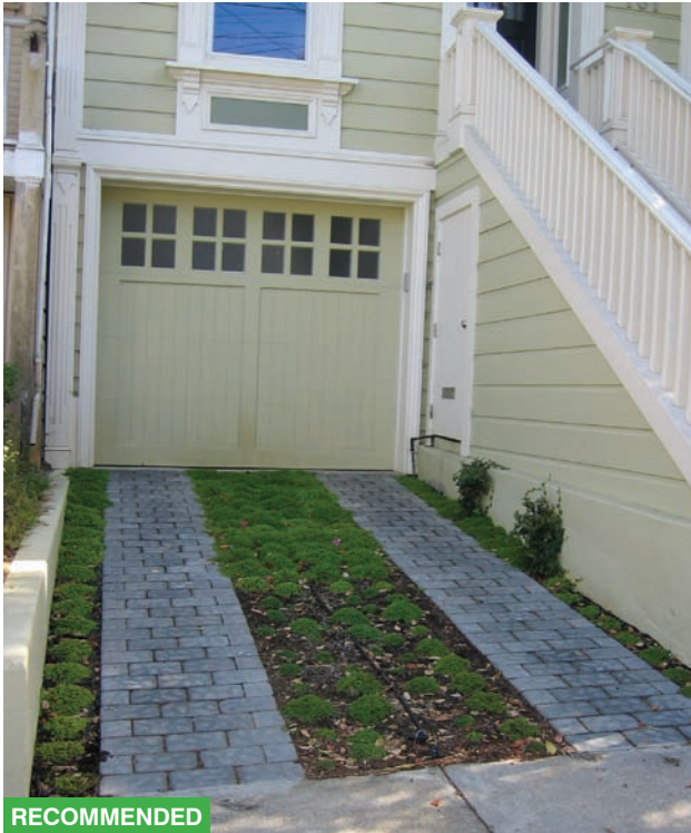
ABOVE LEFT: To maximize landscaping within narrow front setbacks, consider a "Hollywood" driveway, as depicted above, or an open cell paver to allow for grass to grow through and to minimize stormwater runoff.
