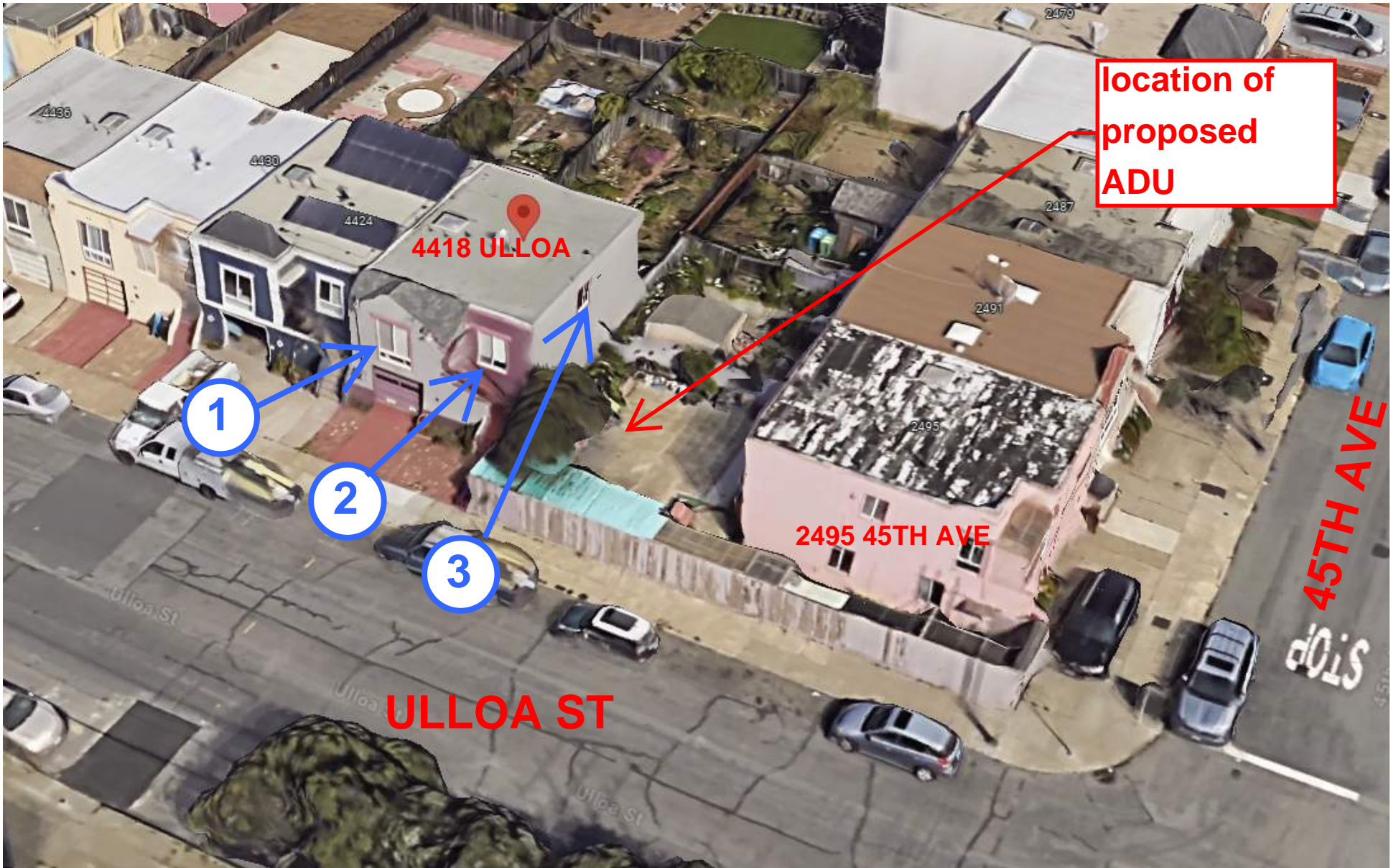
Exhibit 1. ULLOA ST & 45TH AVE. AERIAL FROM SOUTHEAST LOOKING NORTH WEST
