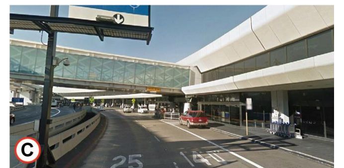
C TERMINAL 3 / AIRTRAIN BRIDGE
