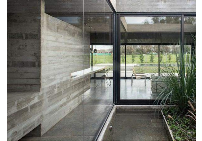
Board form concrete material will be used in outdoor spaces and work to knit the building into Landscape, thus deferring to Historic building
