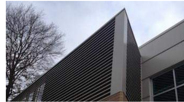
Horizontal louver band at top of concrete walls relate to lower parapet
