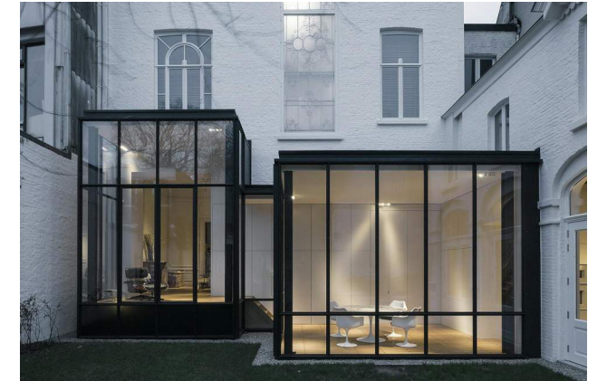
Storefront glazing provides simple transparency to allow Historic Building to be seen from all sides
