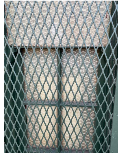
③ EXAMPLE OF PLEXIGLASS INFILL AT WINDOWS
