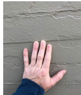
Detail of flush siding
