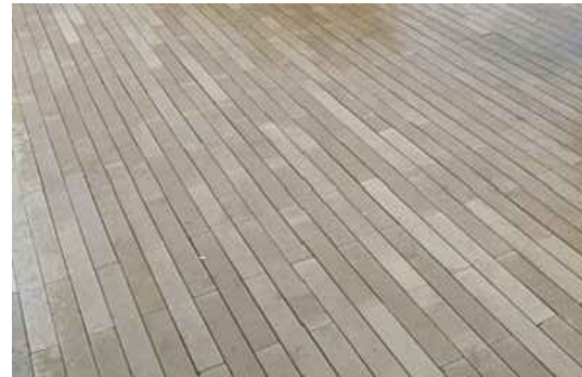
5 SAND-SET CONC. UNIT PAVERS W/ METAL EDGING COLOR: 50% ALMOND, 50% LINEN SIZE: 4" W X 24" L FINISH: GROUND-FACE
