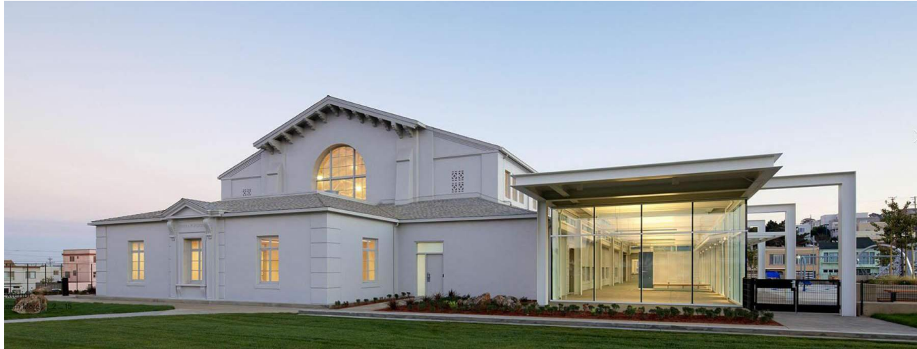
Exterior view of the Palega Recreation Center
