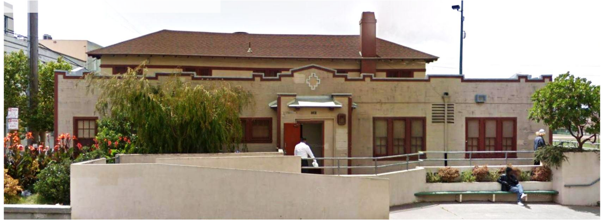
DECKS, RAMPS AND RAILINGS OBSCURE BUILDING ENTRY, ISOLATE FROM PARK
