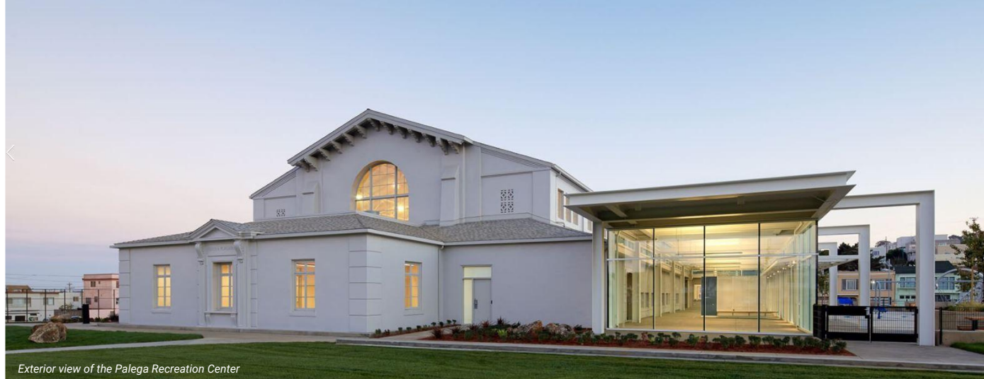
Exterior view of the Palega Recreation Center
