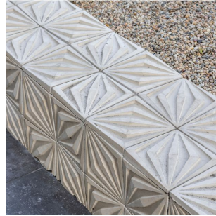
CONCRETE SEAT WALLS WITH TILE VENEER TBD
