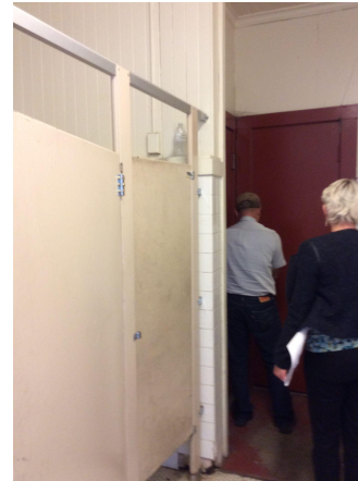
RESTROOMS INADEQUATE IN FIXTURE COUNT + NOT ACCESSIBLE
