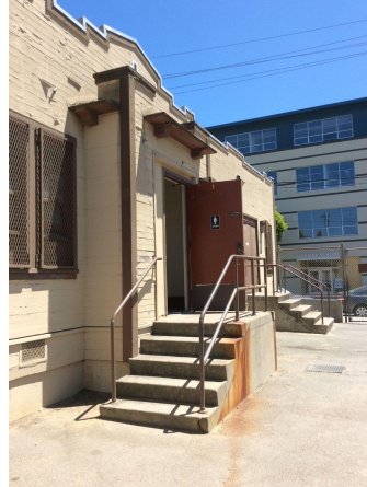
RAMPS & STAIRS ISOLATE BUILDING FROM PARK AND CREATE INACCESSIBLE CONDITIONS
