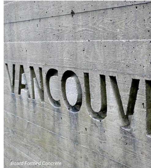
Board Formed Concrete
