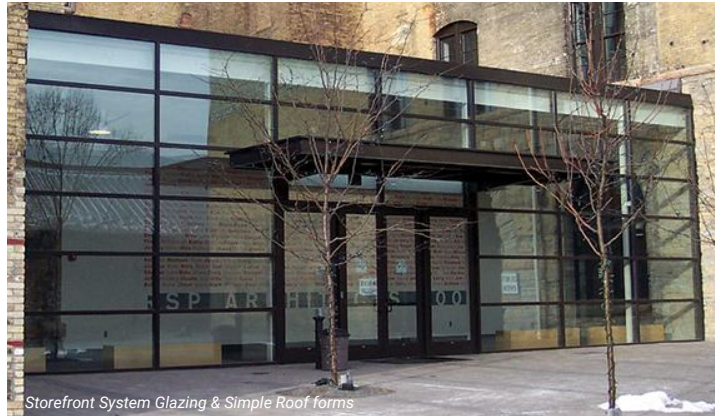
Storefront System Glazing & Simple Roof forms
