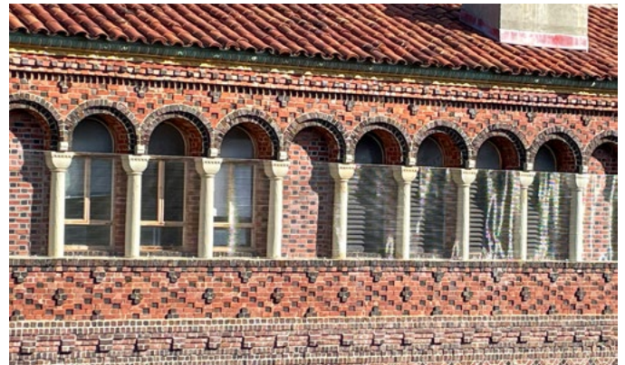
Protective Netting Installed on Historic Buildings
