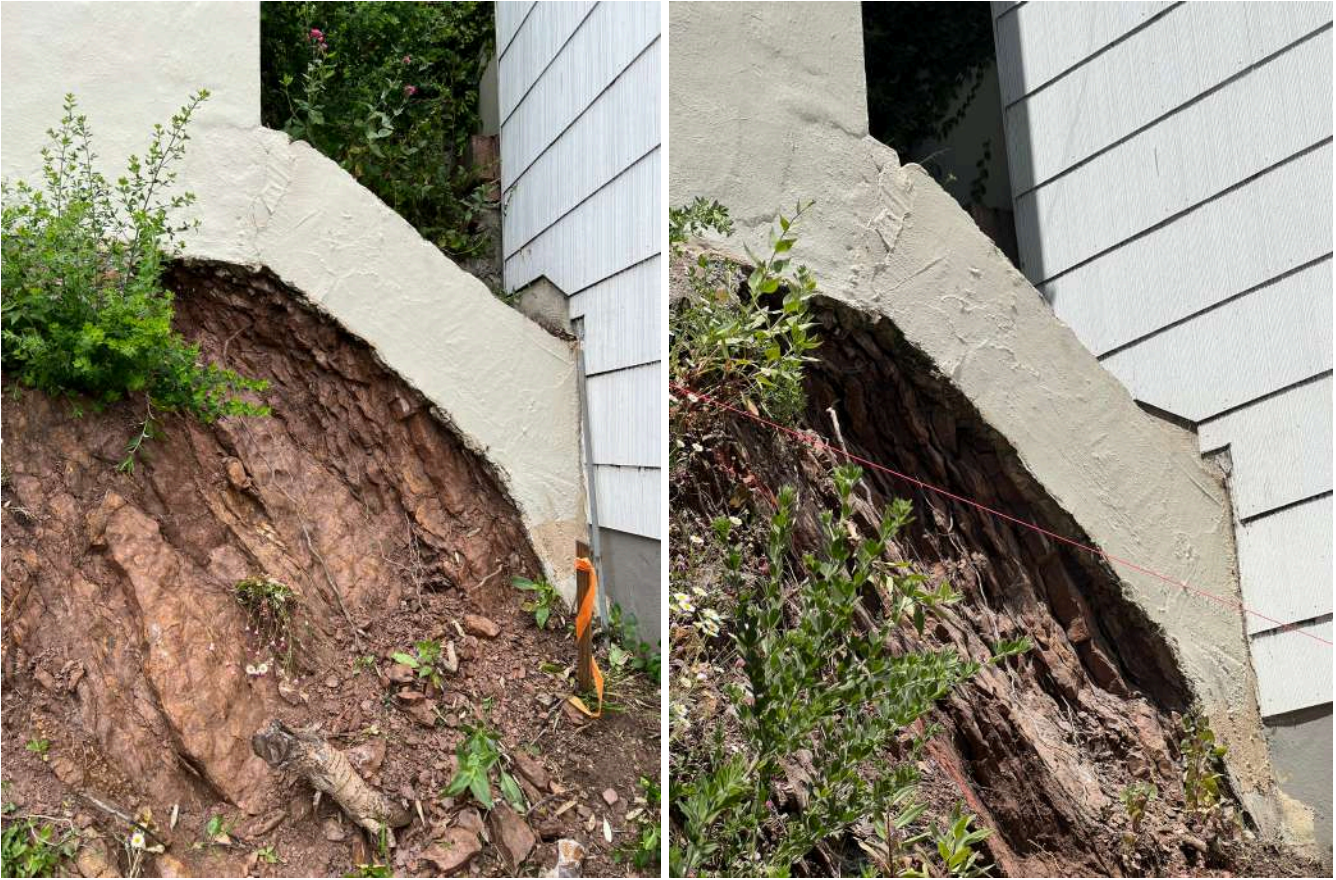
Fig 1. North-West preexisting condition
