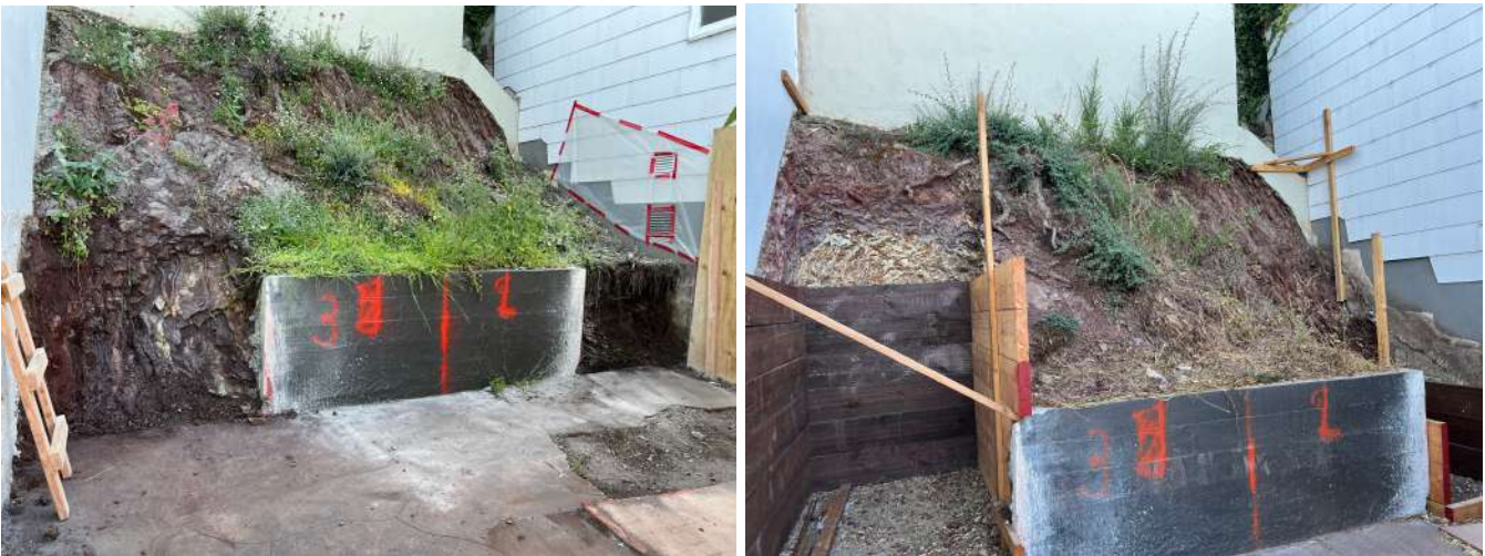
Fig 2. Excavation in sections
